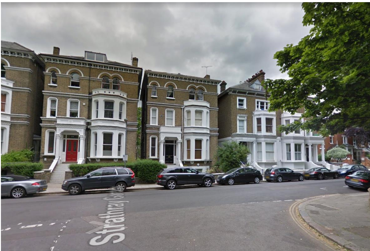
Photo 5 (above): Street view as seen from entrance of Strathray Gardens
