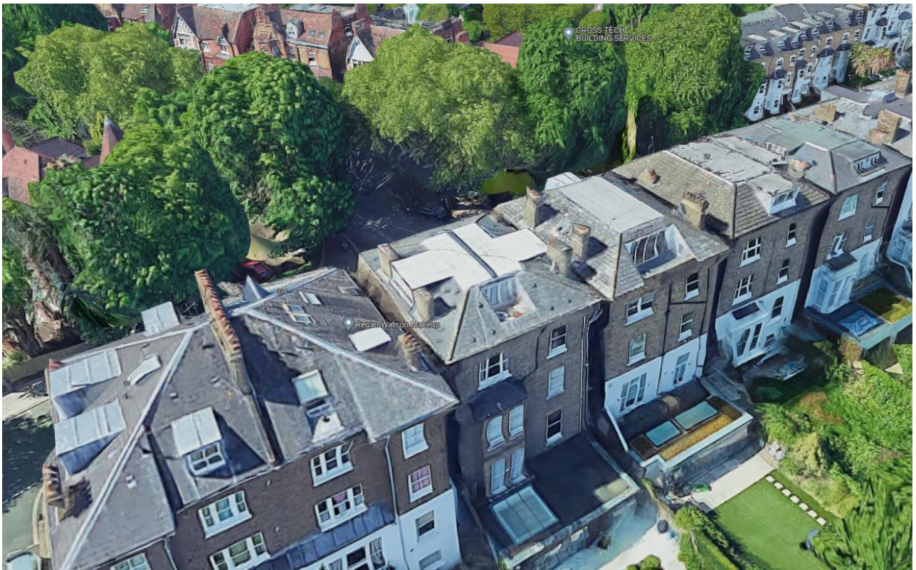
Photo 5 (above): Rear roof terrace
