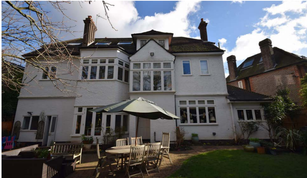
Fig 5: View of rear elevation showing mismatched bay and stair outrigger
