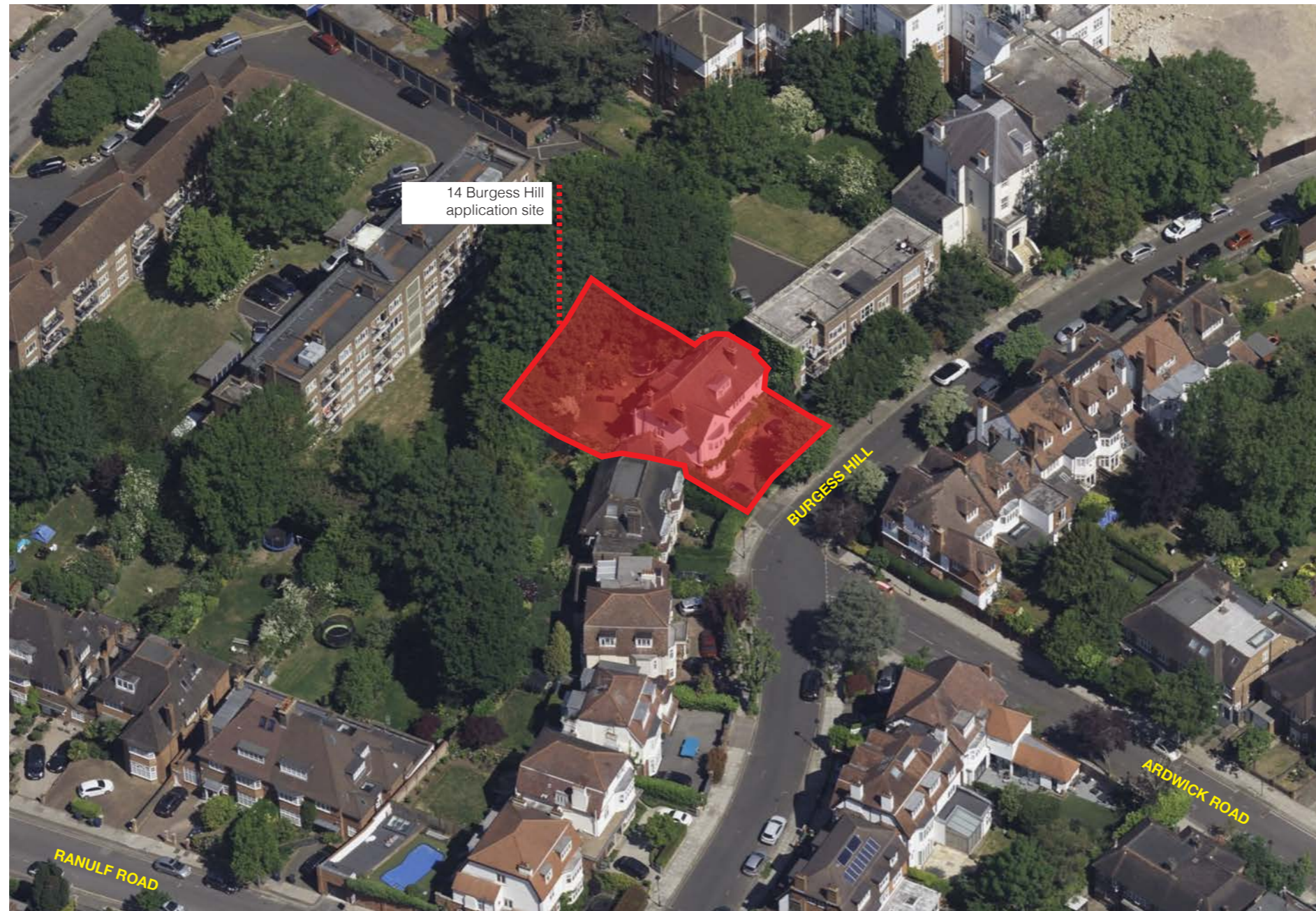
Fig 2: Aerial view of site and surrounding context
