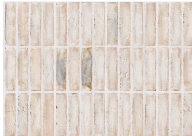
Fig 14: Example photo of soldier course brickwork to be used in header element - complementary colour, texture and variation
