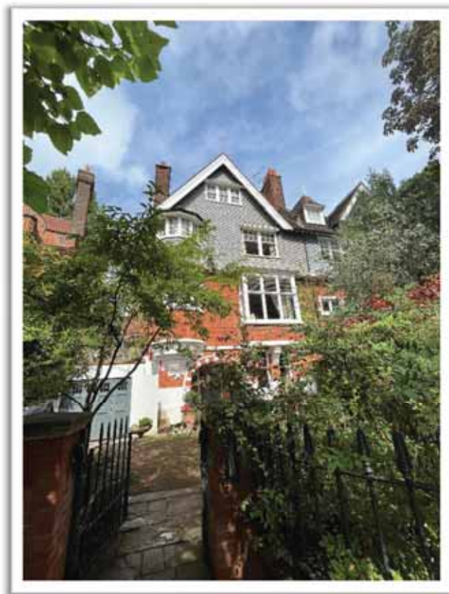
Image 5: Front elevation to No. 3 Gainsborough Gardens
