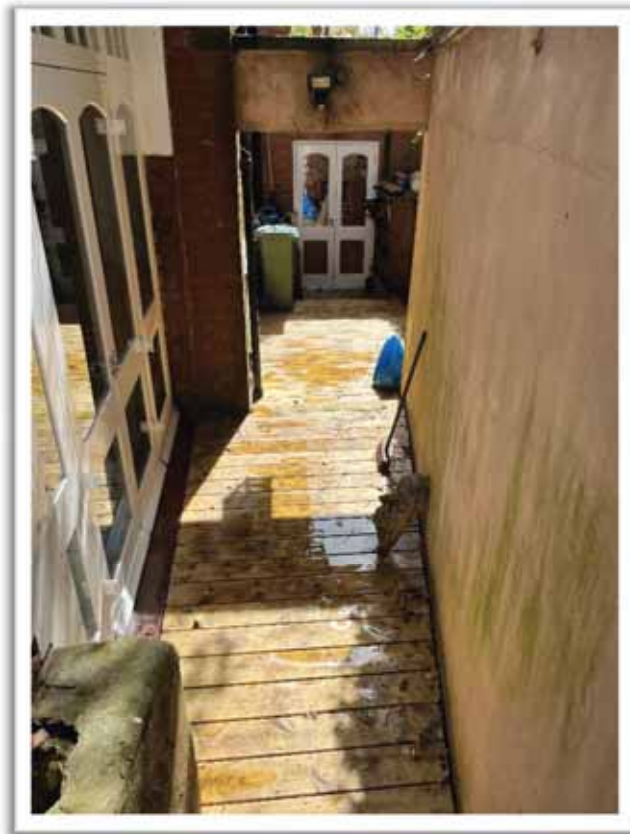
Image 13: Existing narrow area proposed for infill extension
