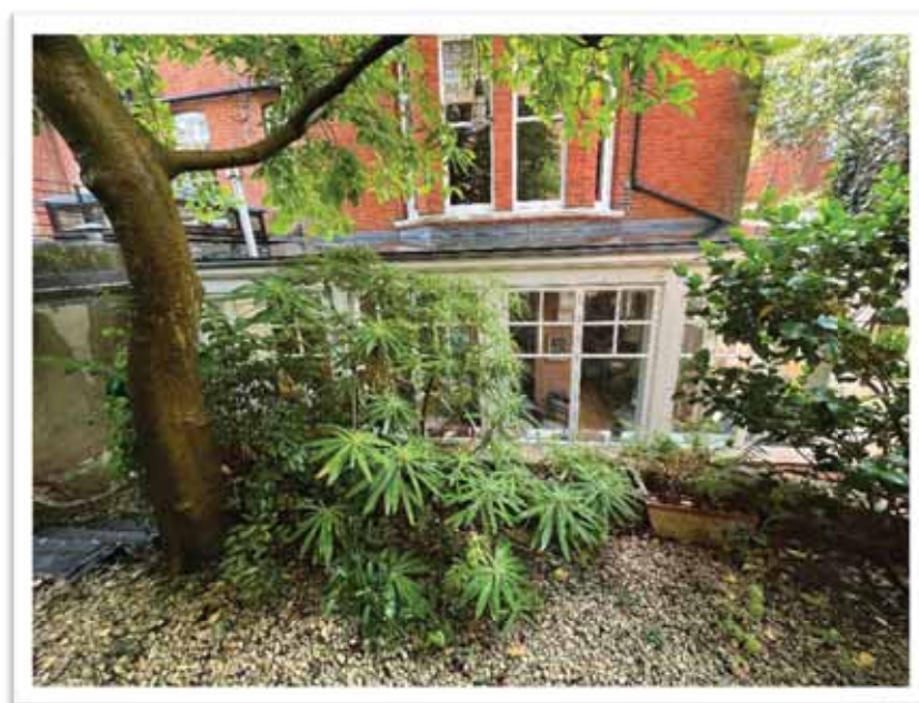
Image 12: Existing rear lean-to extension
