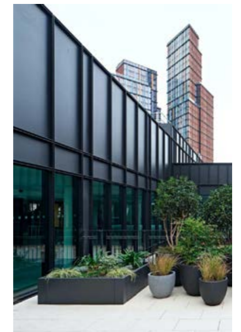
Reference image of metal cladding
