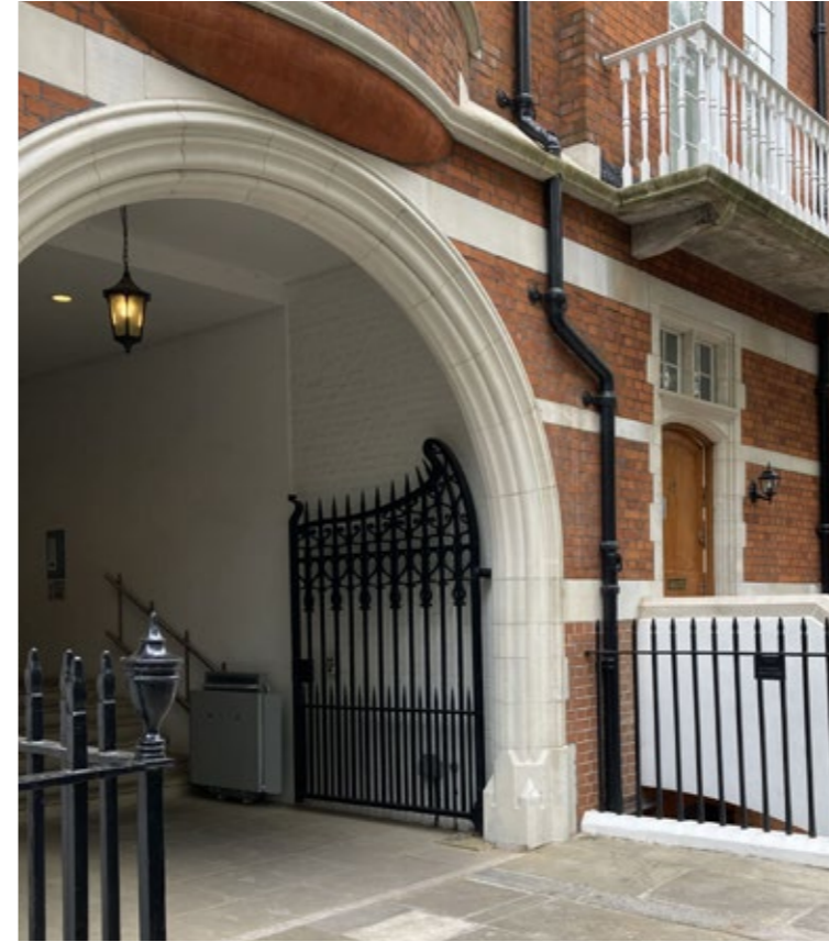
Existing Stonework + Railings on Bedford Court Mansions
