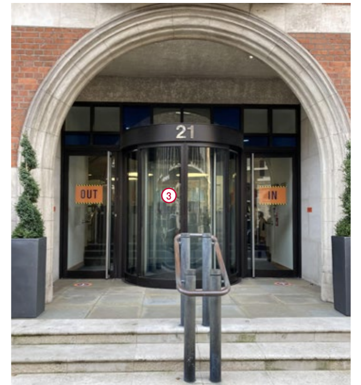
Existing main reception entrance
