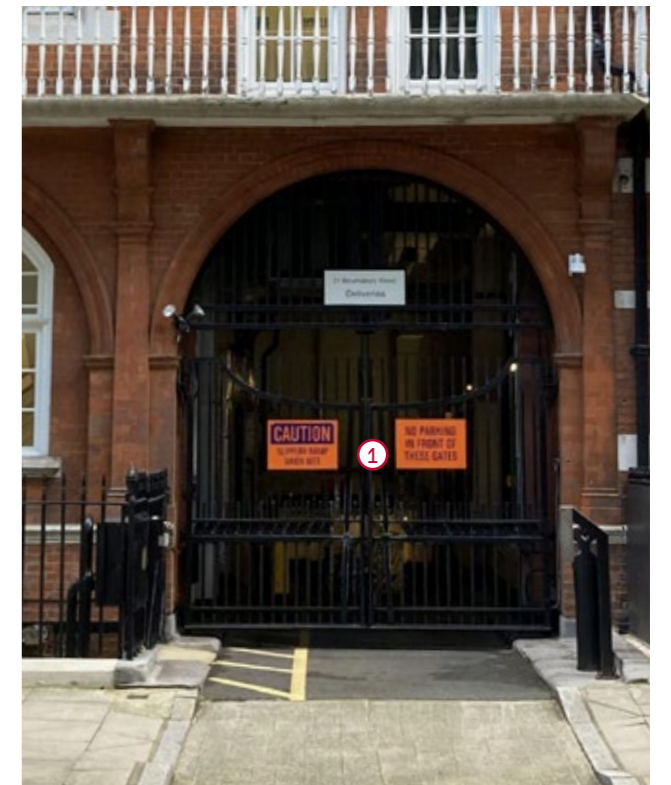
Existing car & cycle store entrance
