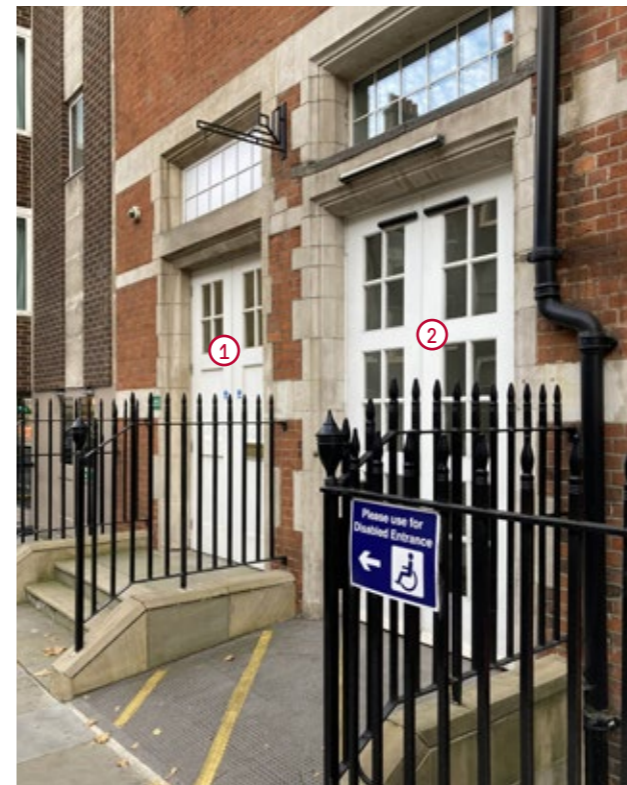
Existing accessible entrance & fire egress
