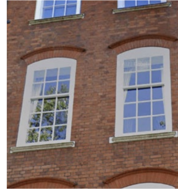
Timber Frame Sash Windows
