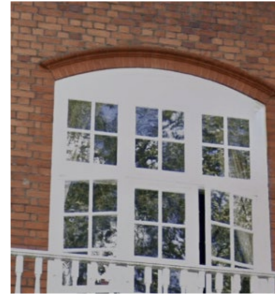
Timber Frame Sash Windows
