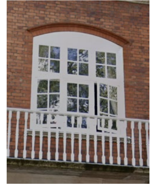
Timber Frame Casement Windows
