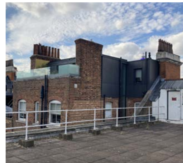
6th floor view with flank wall and obscured windows
