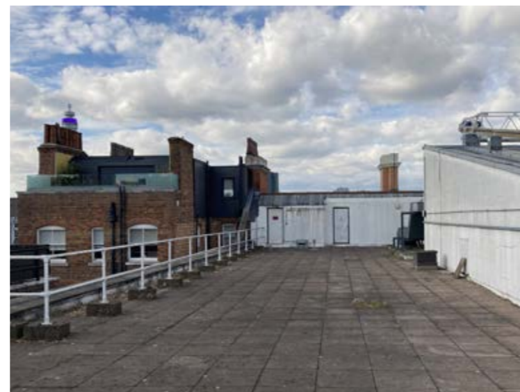
View from existing roof level (L06) towards Bedford Court Mansions
