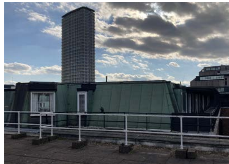
View from existing roof level (L06) towards Bedford Court Mansions
