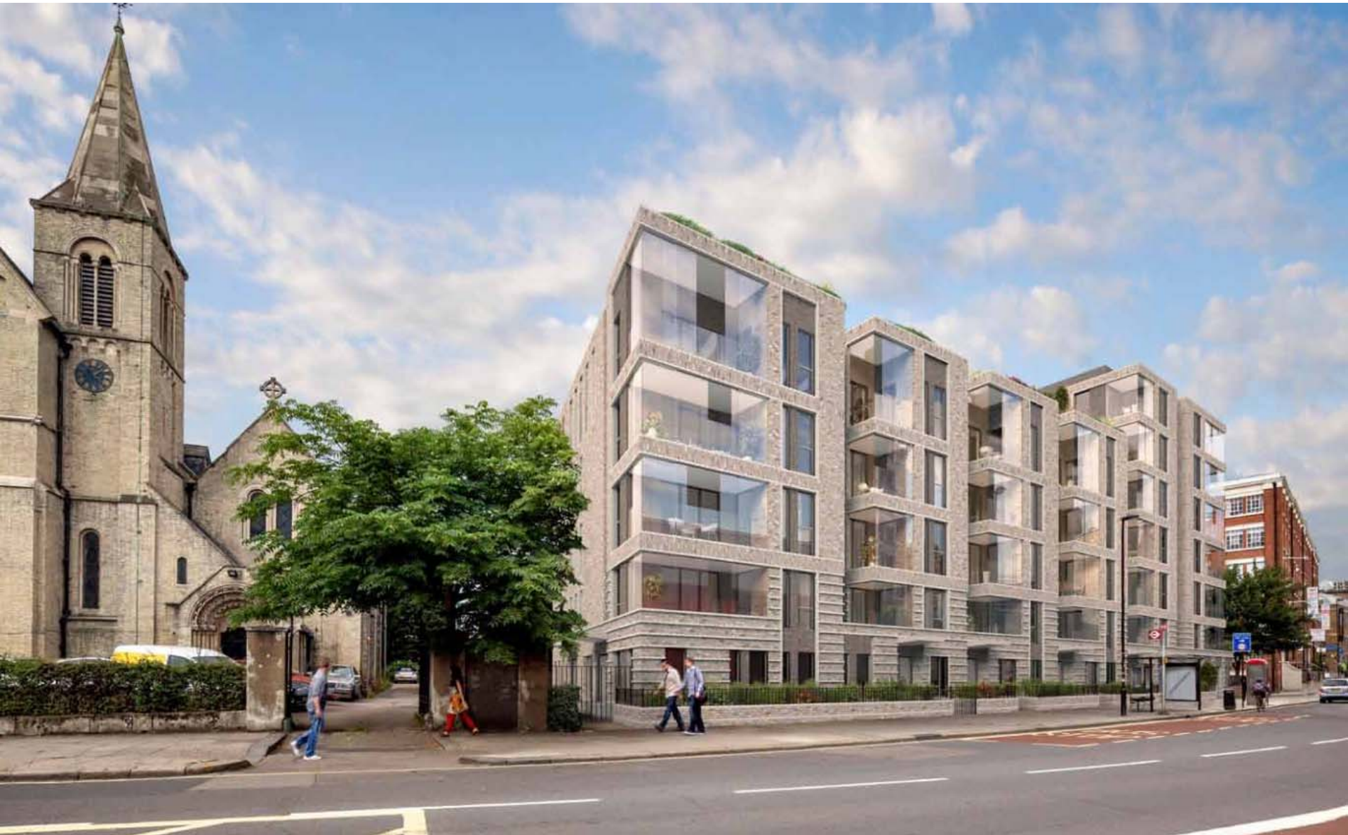
Residential building: Highgate Road elevation view
