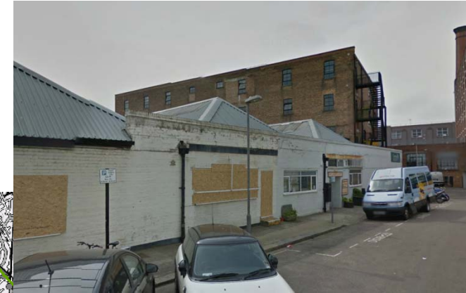
Greenwood Centre – learning and other disabilities day care service, 1,900 sqm (part-vacant and part occupied by the Camden Society)
