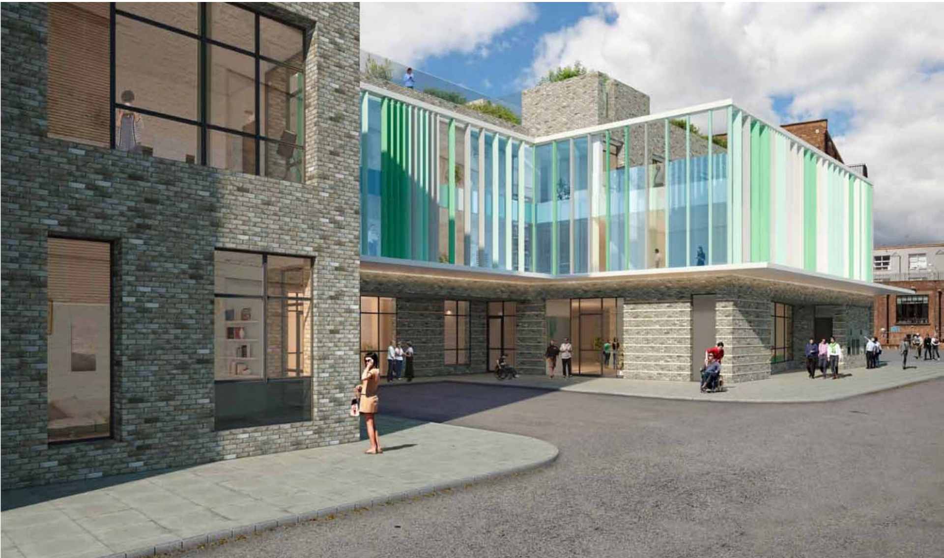
Greenwood CIL: View from Greenwood Place showing drop-off/delivery bay and entrance area
