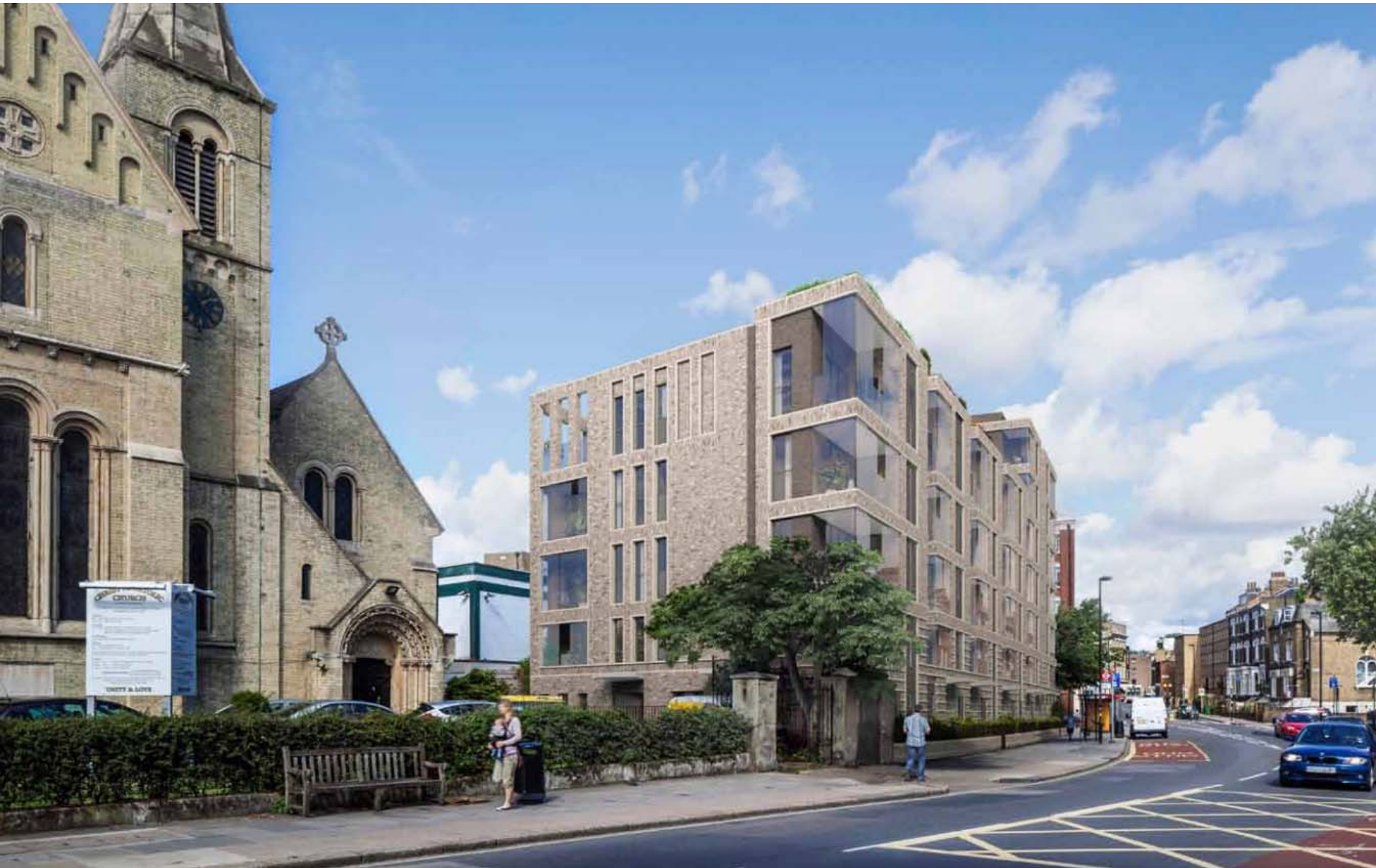
Residential building: South elevation view
