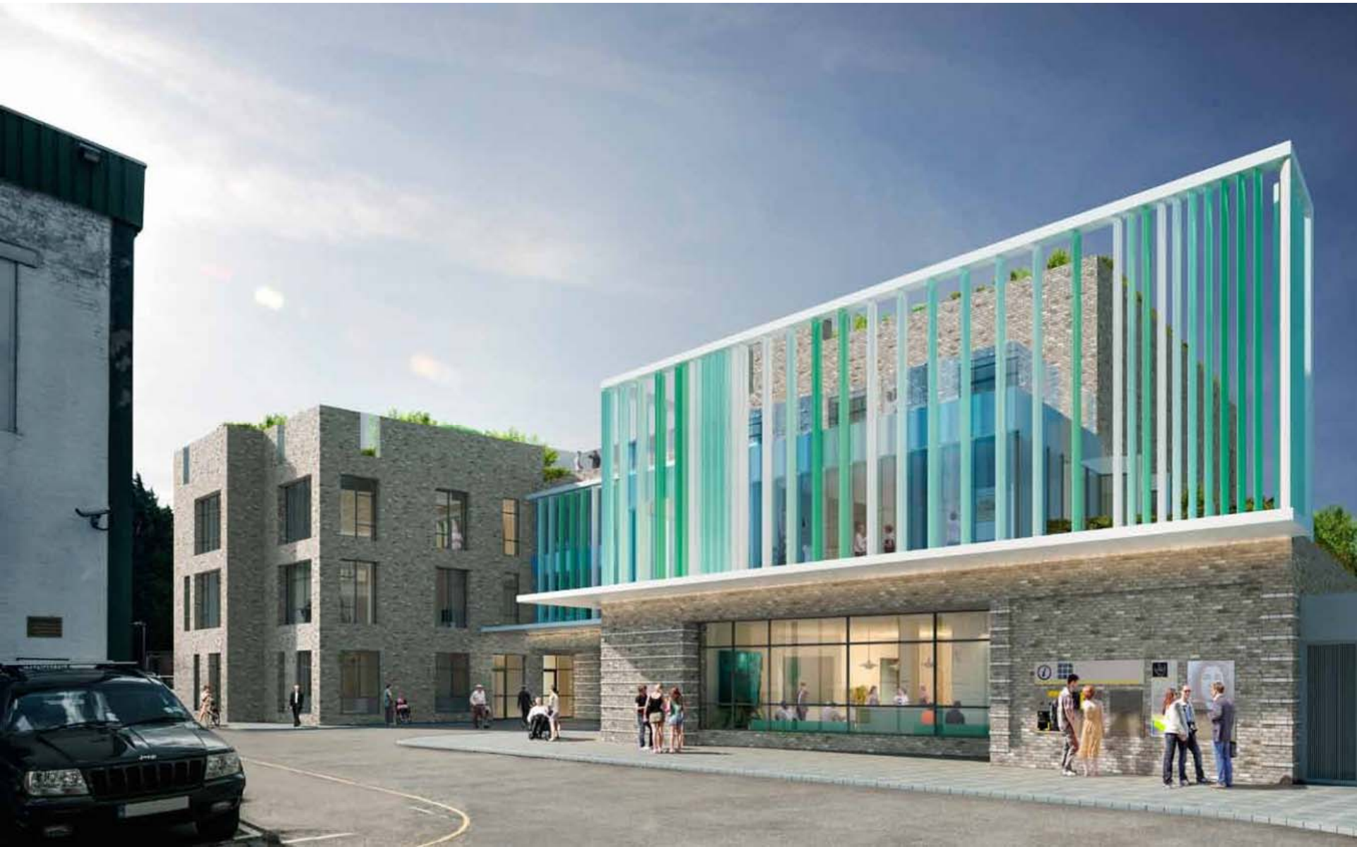
Greenwood CIL: View from north on Greenwood Place
