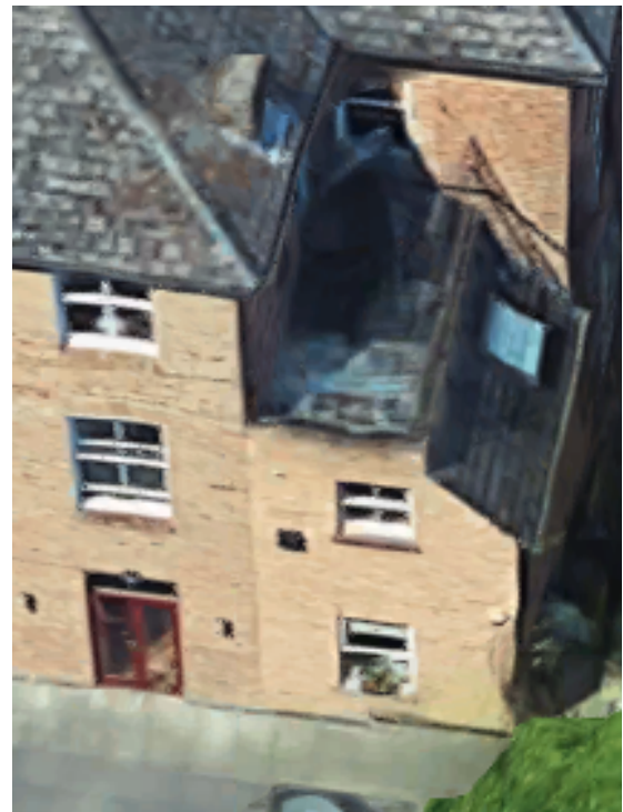
68 Priory Road - Aerial view of first floor rear extension
