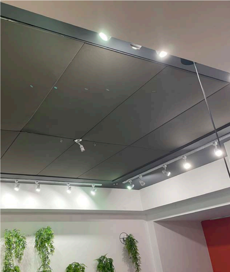
Existing false ceilings in small retail unit.
