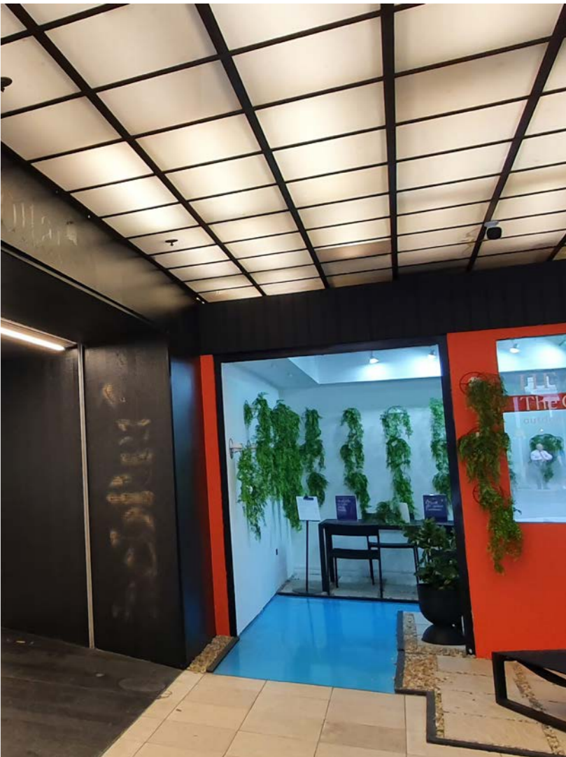
Existing lightbox ceiling and segregated retail units.
