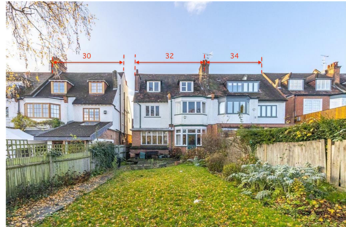
Existing rear elevation to nos. 30-36 Crediton Hill
