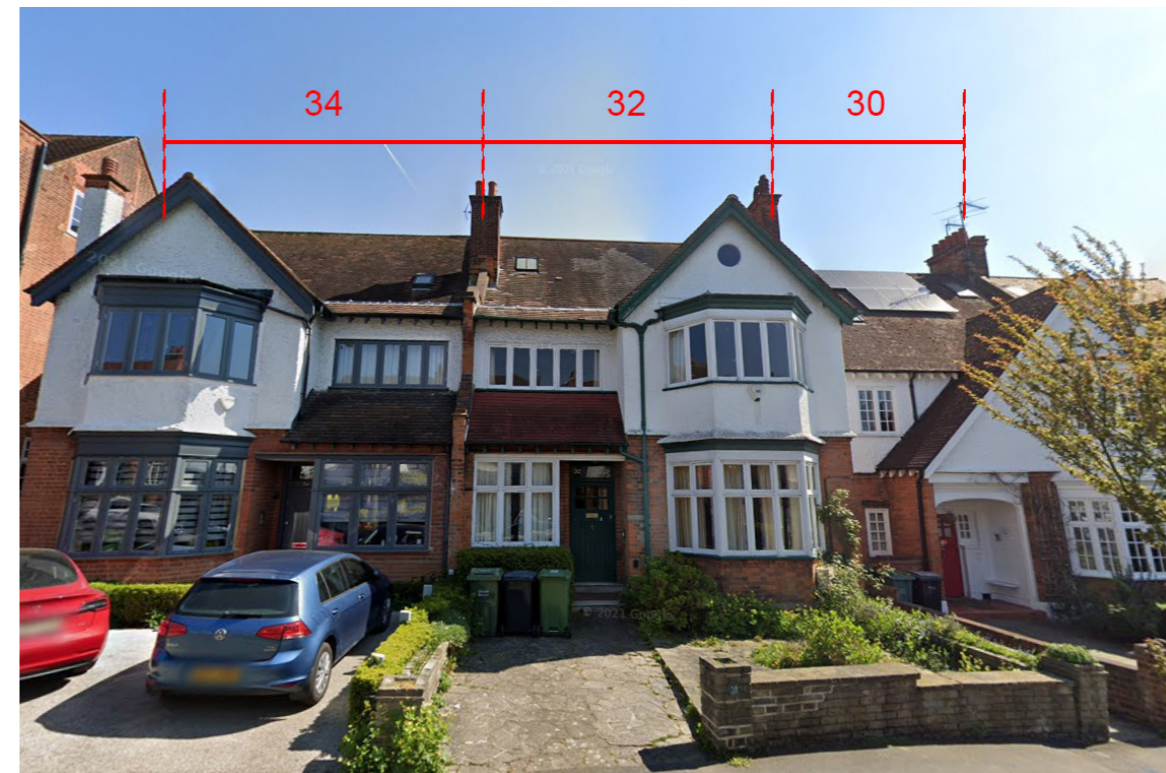
Existing entrance elevation to nos. 30-34 Crediton Hill
