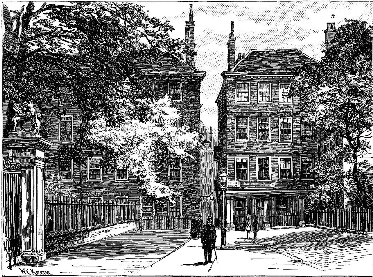
Fig 5 – Engraving of Field Court c.1890 looking east toward rear of 1 Gray's Inn Place (left) and 10 South Square (right). Note stone doorcase to former building on right (4 Field Court)
