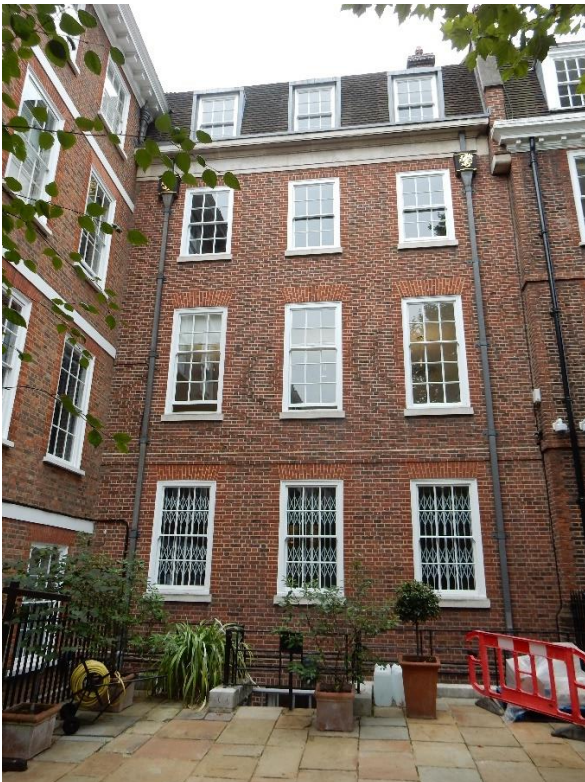
Fig 3 - North elevation of 10A South Square facing onto Field Court
