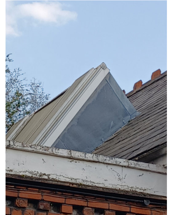
Detail of slate roof and north roof light opening to No.12 with later frame inserted and modern detailing, 2022 (Purcell).
