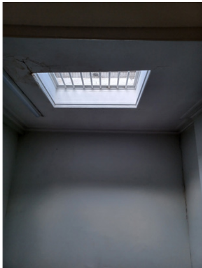
Original rooflight opening to 'rear room' with modern skylight fitted. 2022 (Purcell)
