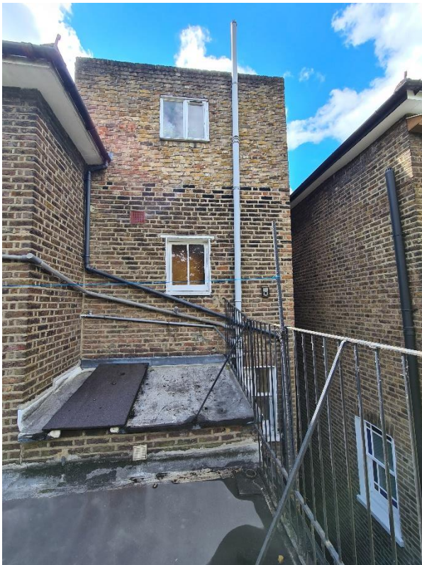
Rear elevation showing limited windows and proposed casement windows to be replaced with sash windows and Juliette Balcony
