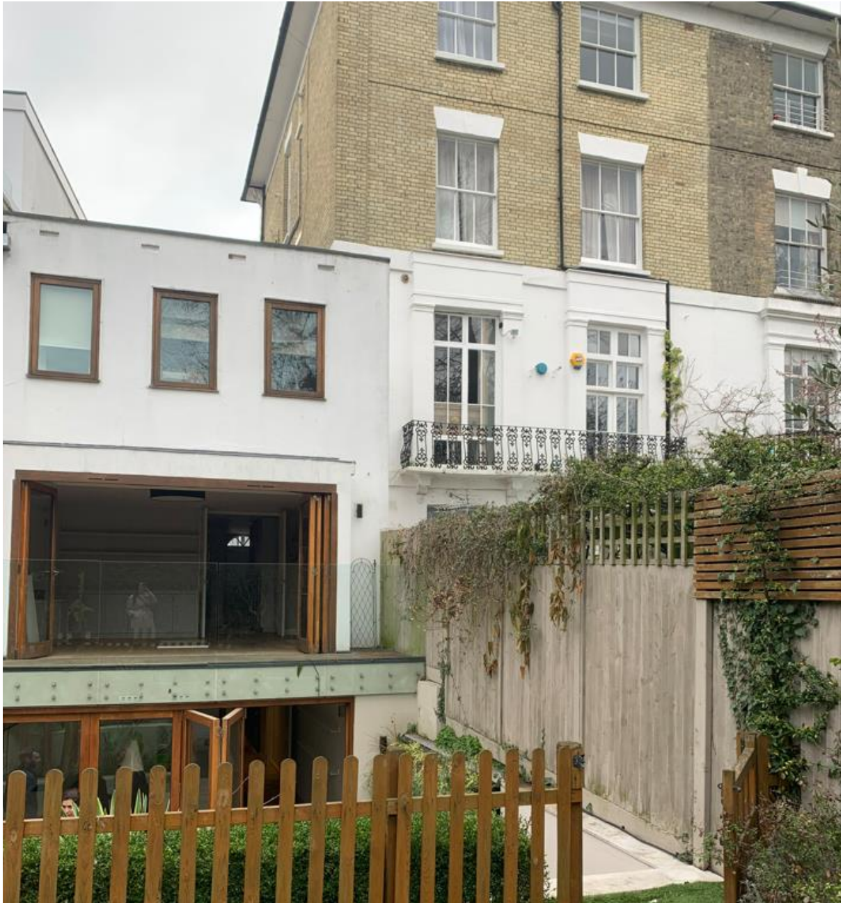
Photo 6 (above) – Rear façade and view towards no 26.
