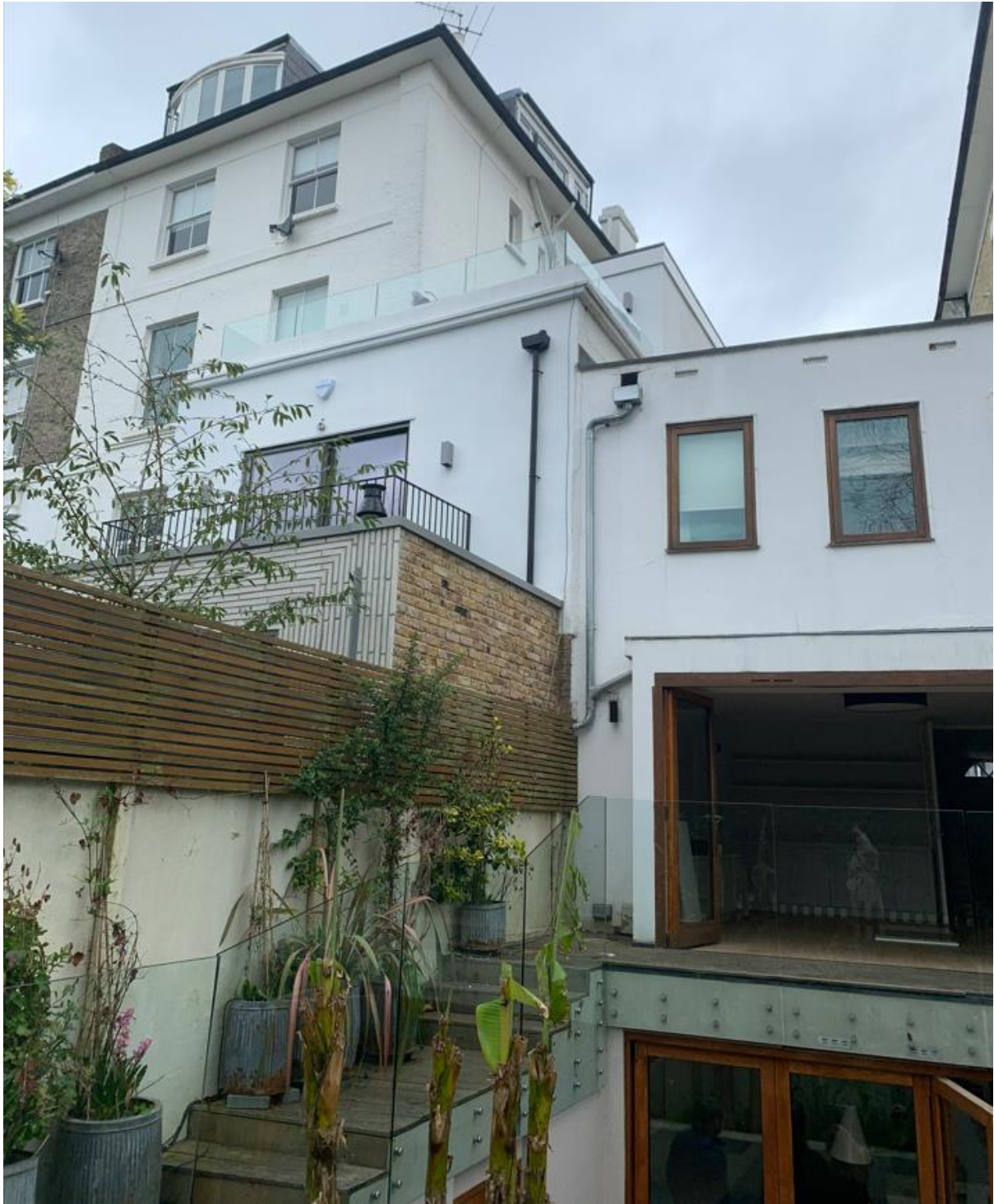
Photo 5 (above) – Rear façade and view towards no 24.
