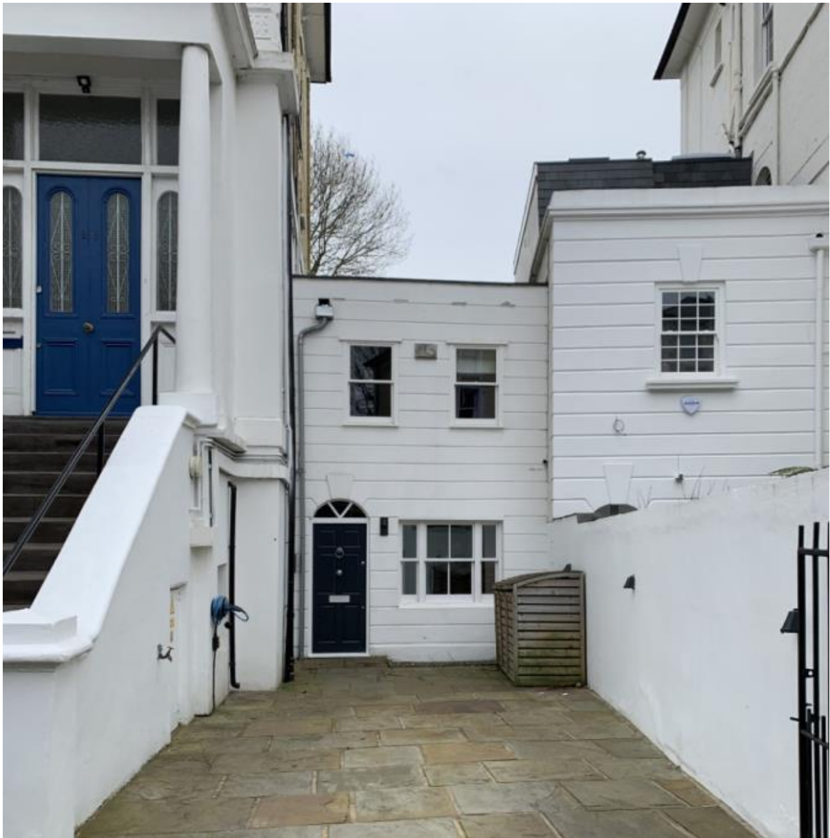
Photo 3 (above): Front façade as seen from street
