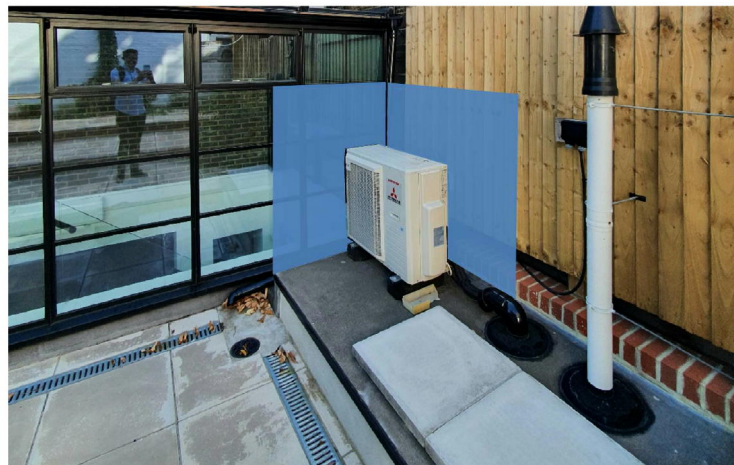
Figure 6.1: Location of proposed acoustic panels (to extend behind condenser unit)
