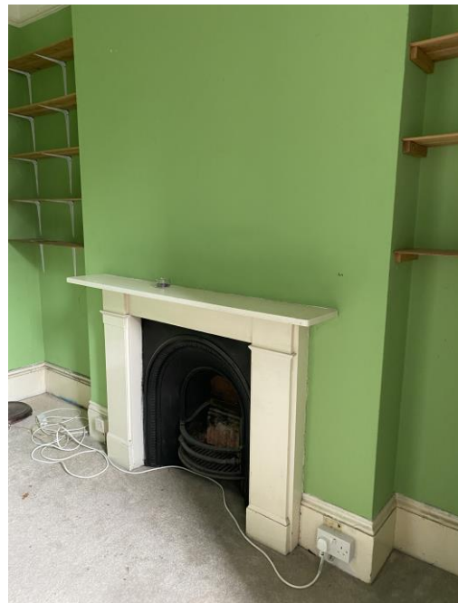
Figure 14: Original fireplace to rear room and original skirting.
