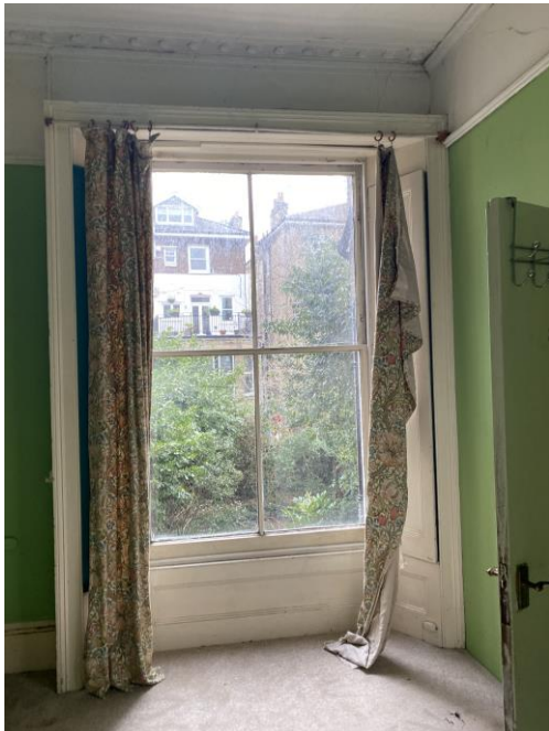
Figure 12: Rear room window with lining and shutters.
