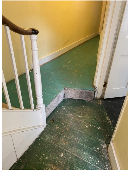
Figure 20: Platform in lower ground floor hallway.
