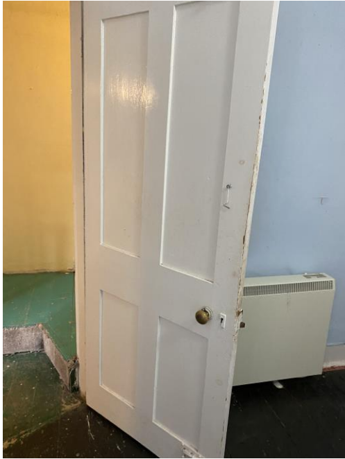
Figure 24: Door to rear room with typical details
