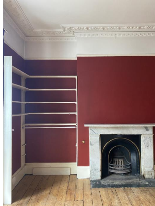
Figure 10: Cornice and fire surround detail, front room.
