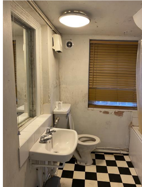
Figure 26: Rear bathroom, lower ground floor.
