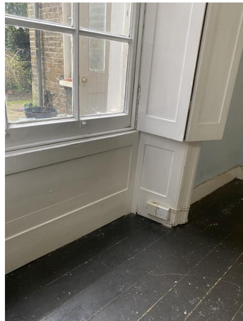
Figure 23: Original rear window details.
