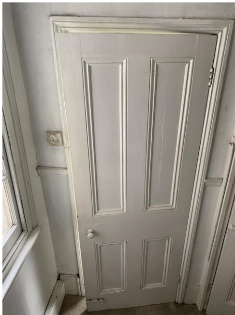
Figure 15: Door to rear bathroom with moulded detail to panels on the house side and simple four panels on the inside.
