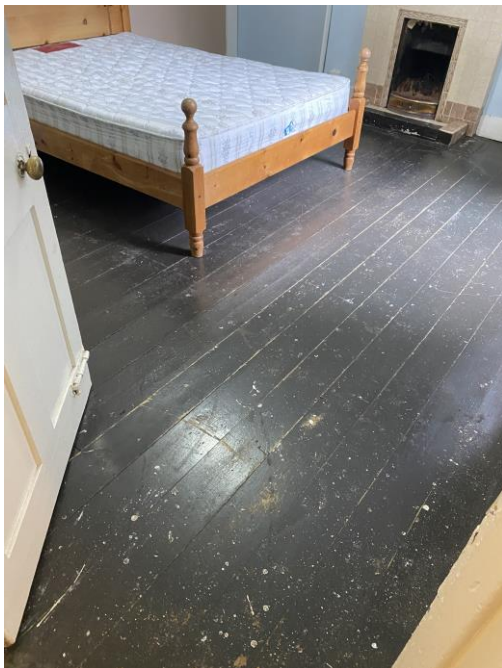
Figure 25: Rear room floor finish.
