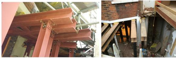
Figure 1 Example of needling to existing wall
