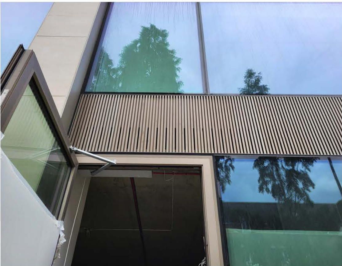
Existing external photograph showing decorative 'louvre' panels
