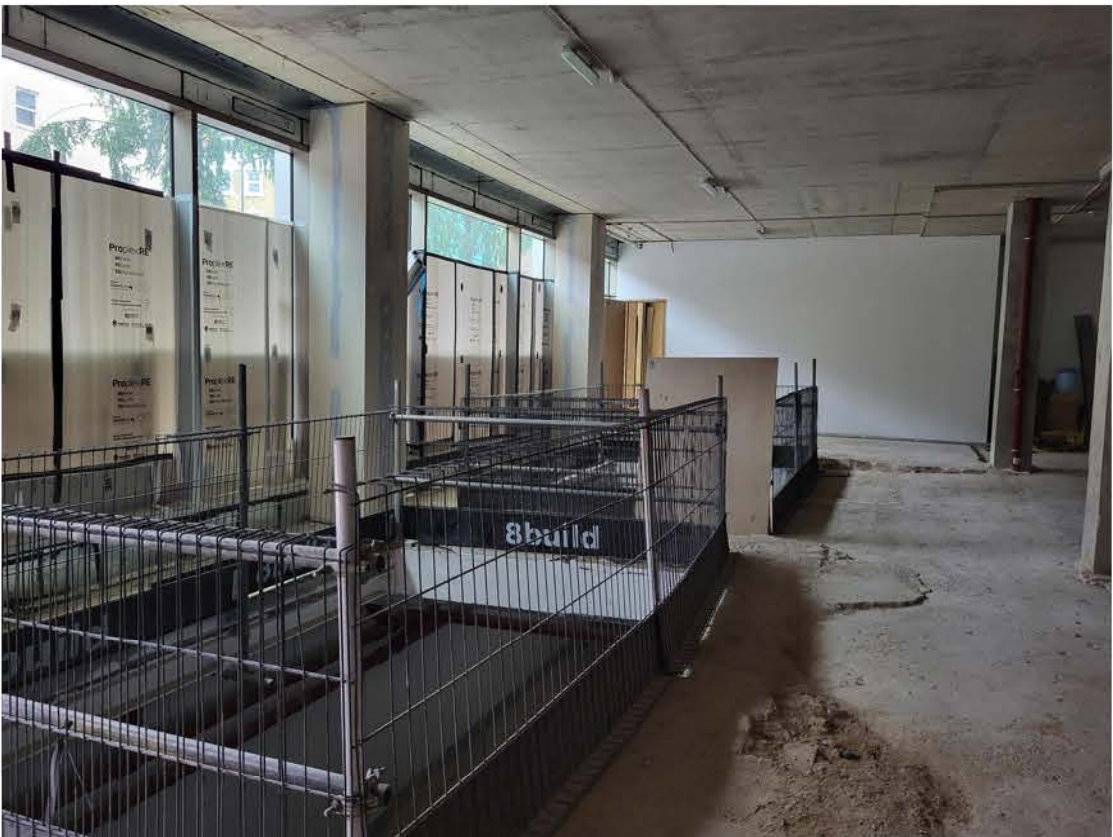
Existing internal photograph showing decorative 'louvre' panels blocked up
