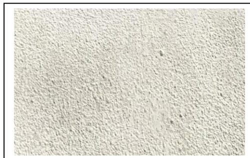
Figure 2. Appearance of render with rough cast finish painted white.
