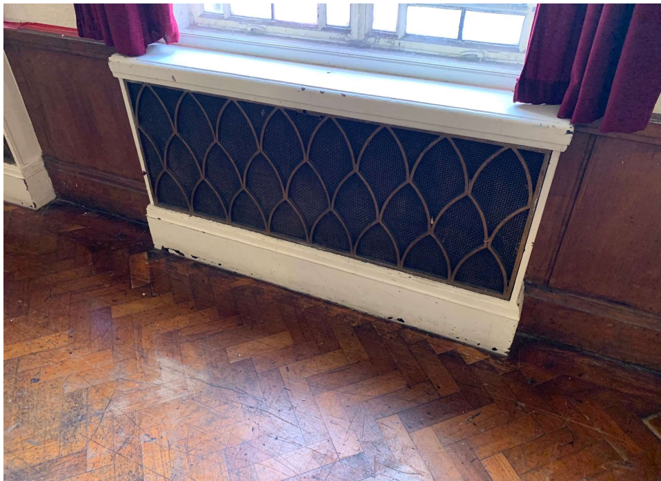
Photo 002 - Grille over existing radiators
