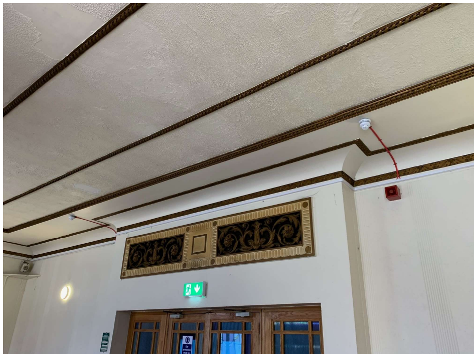
Photo 006 - Showing iron grille, ceiling plaster and cornice
