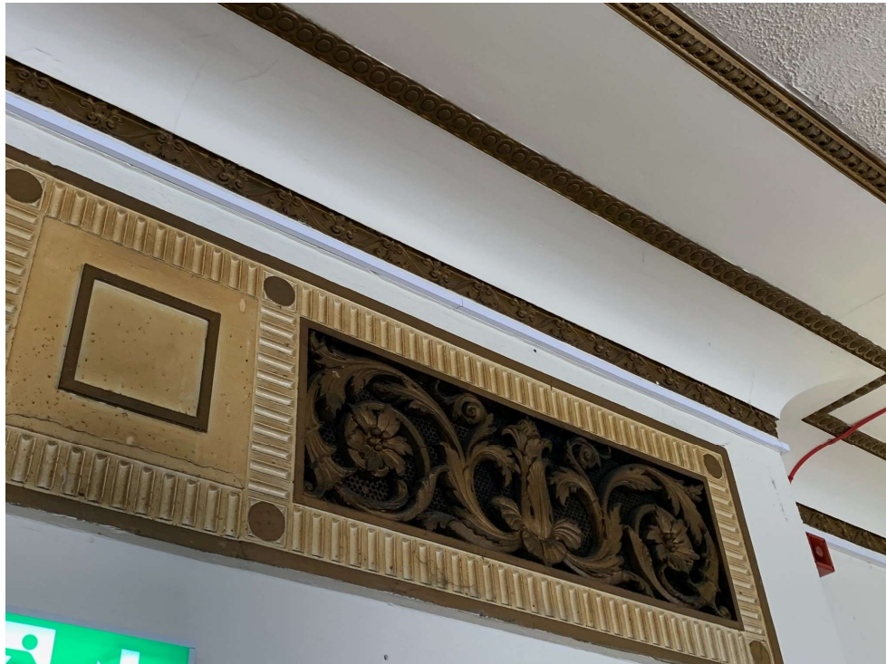
Photo 001 - Iron grille over main entrance door to existing tearoom
