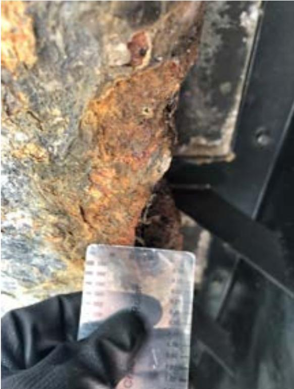
**Photo 7:** Full thickness section loss of bottom flange of canal side edge beam towards west abutment
