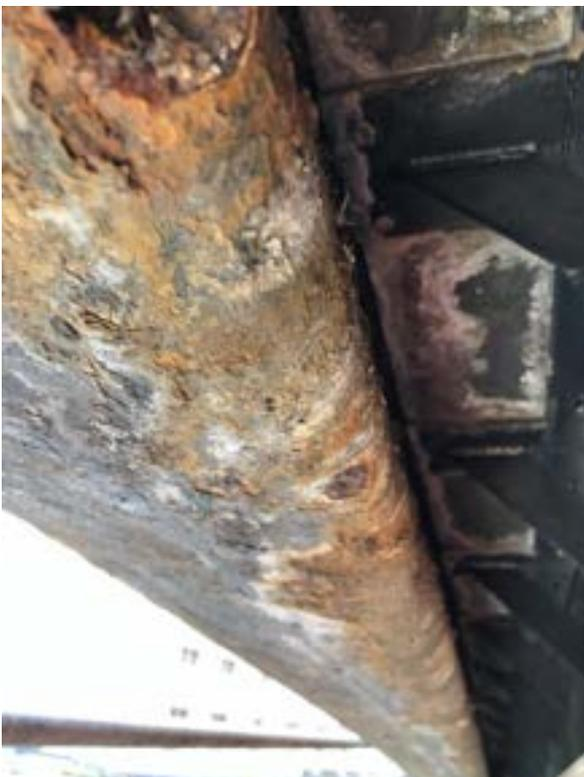
**Photo 3:** Delamination of southside edge I girder
