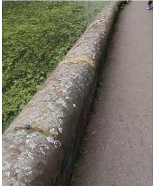
**Photo 30:** Algae on the west ramp parapet.
