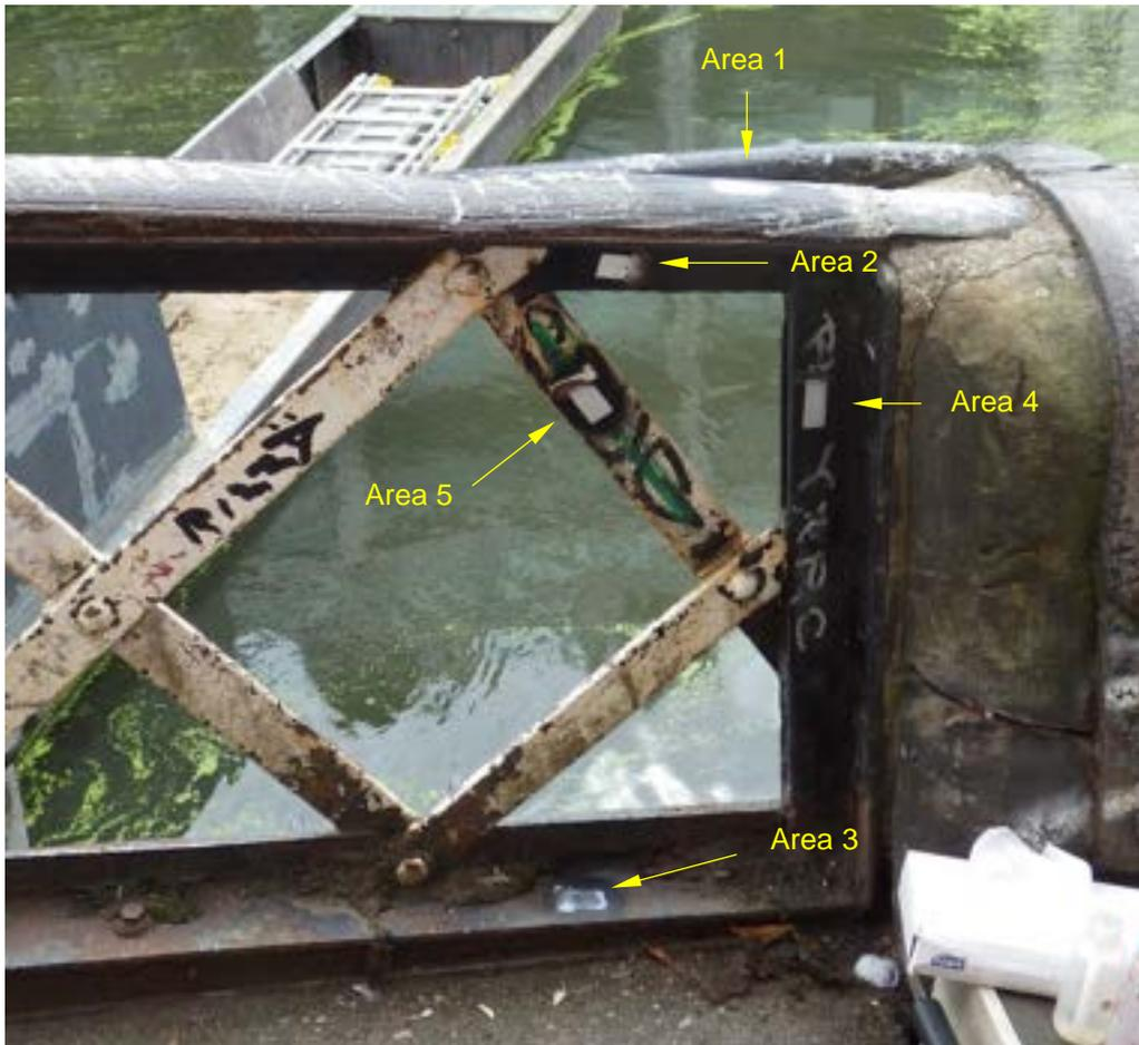
Figure 1: Overview of Areas 1 to 5 showing locations of RM testing and paint samples.
