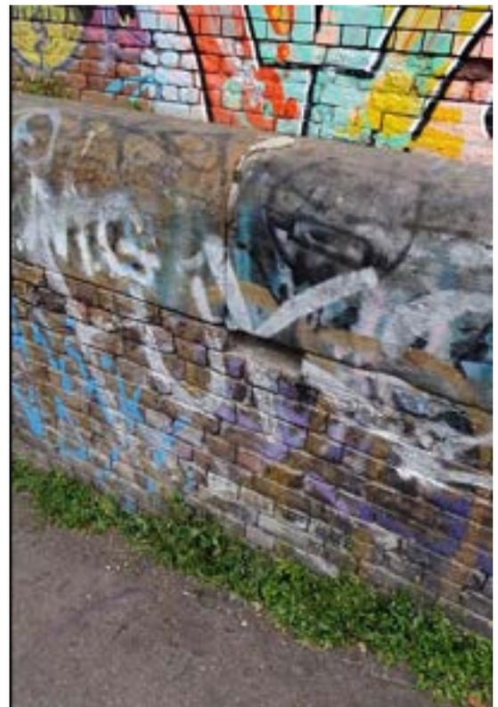
**Photo 28:** Loss of mortar and brick to the boundary wall.
