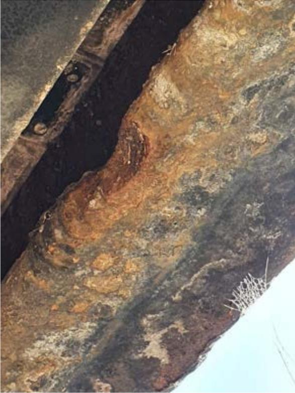
**Photo 5:** Full thickness section loss of bottom flange of canal side edge beam
