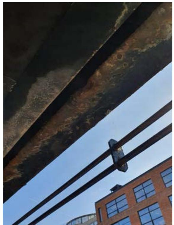
**Photo 4:** Full thickness section loss of bottom flange of canal side edge beam
