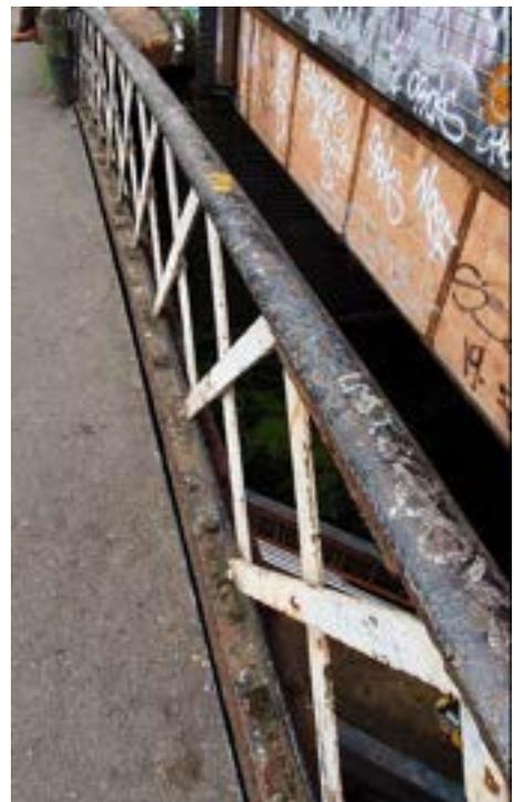
**Photo 38:** Alignment of parapet has moved away from the deck structure
