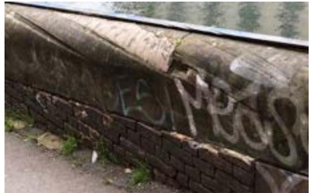
**Photo 26:** Minor graffiti and loss of mortar to the ramp parapet
