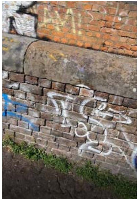
**Photo 24:** Loss of mortar to the boundary wall on the east ramp
