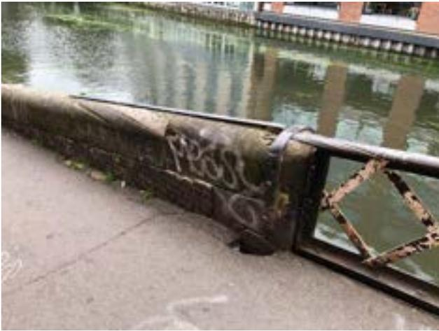
**Photo 25:** stapled connection - canal side parapet
