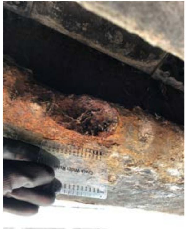
**Photo 6:** Full thickness section loss of bottom flange of canal side edge beam towards west abutment
