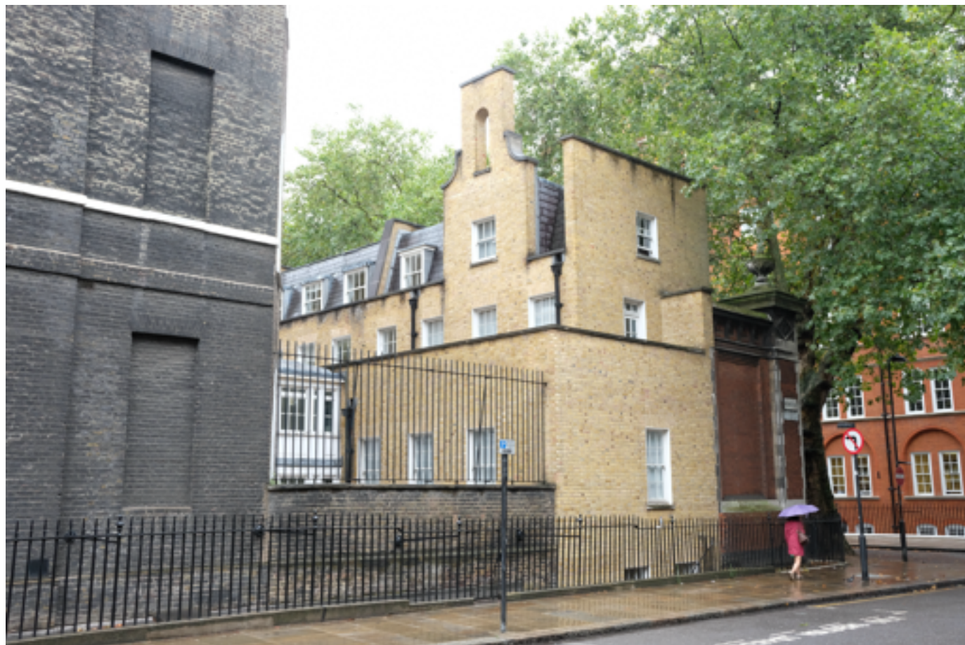
The paler brick was constructed in 1980s. The proposed air vent locations are to be added to this newer brick, therefore the new vents will have no impact on the historic 1890s fabric.
