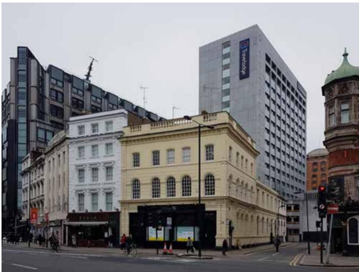
Figure 1 View of existing site from West Central Street
