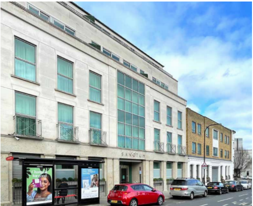
SOUTH ELEVATION VIEW OF BELSIZE ROAD
