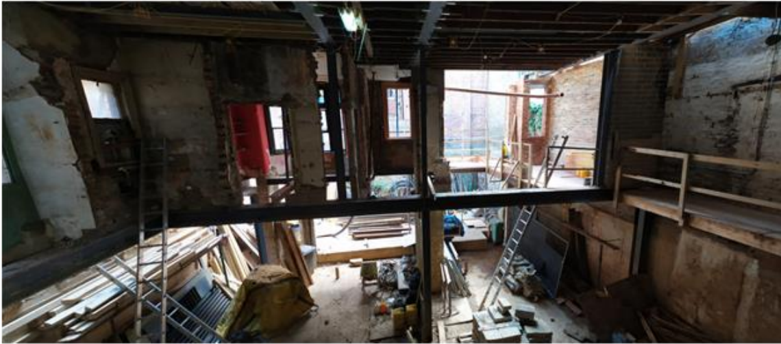
Figure 1. View of excavated basement
