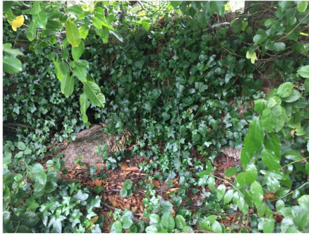
Figure 4 - Retaining party fence wall to rear of property taken from No.30 facing the garden
