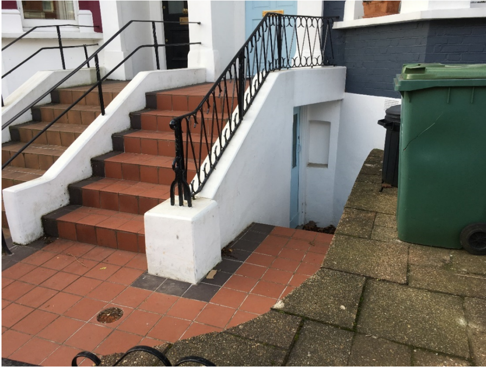
4. View of front stairs (to be retained)
