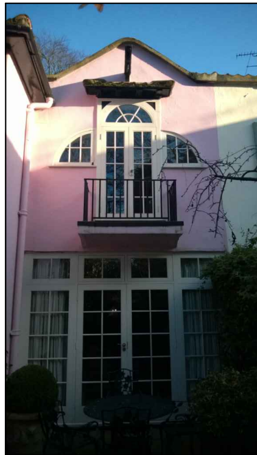
DP7- Front Elevation - View NE
