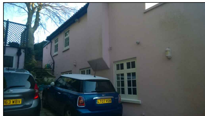
DP8- NW Elevation - View E
