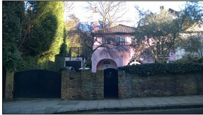
DP1- Building Frontage - View NE
