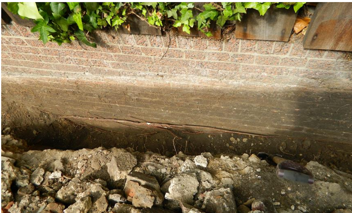
Figure 6. Root thought to be from the neighbour's cypress growing along face of boundary wall foundations.
