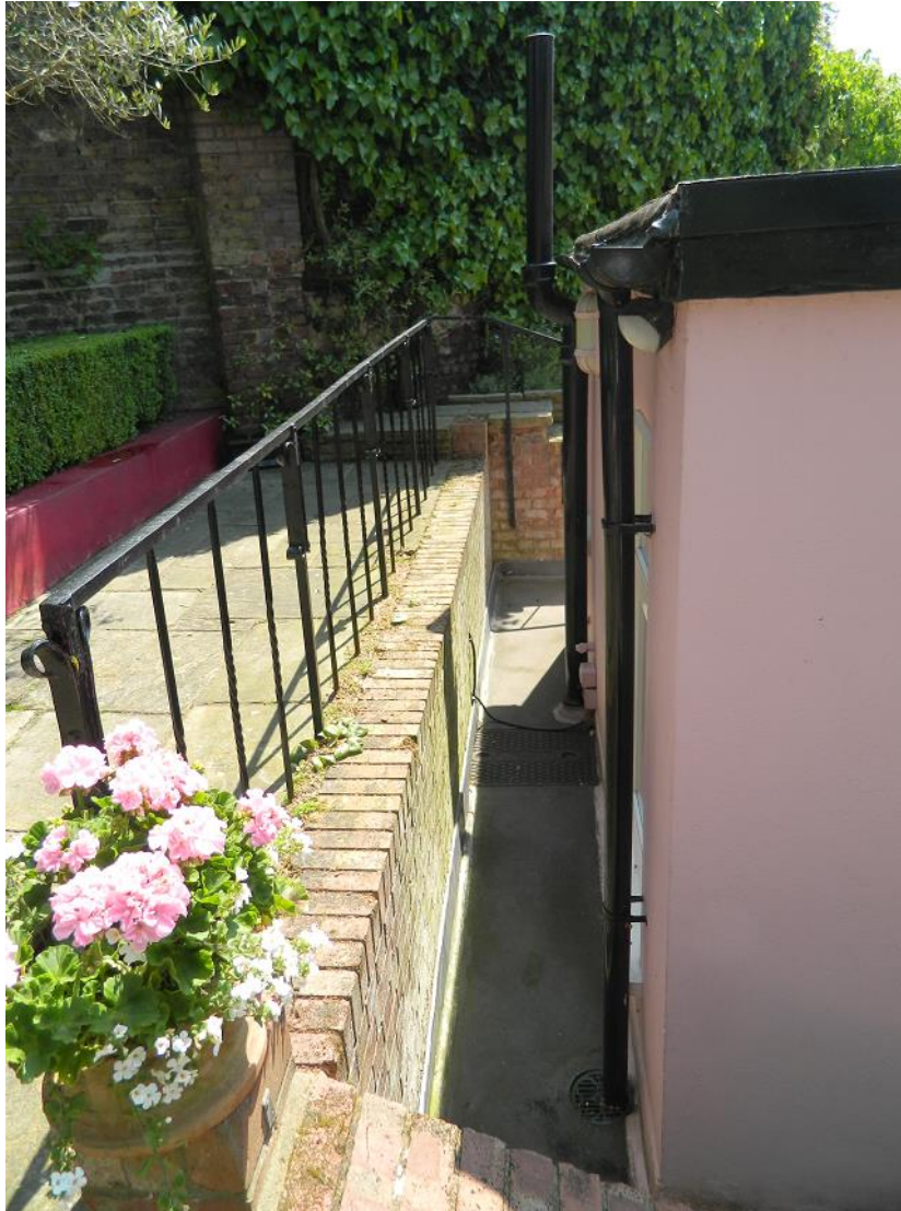
Figure 8. Retaining wall to the rear of the property which marks the edge of proposed development which will act as a root barrier.
