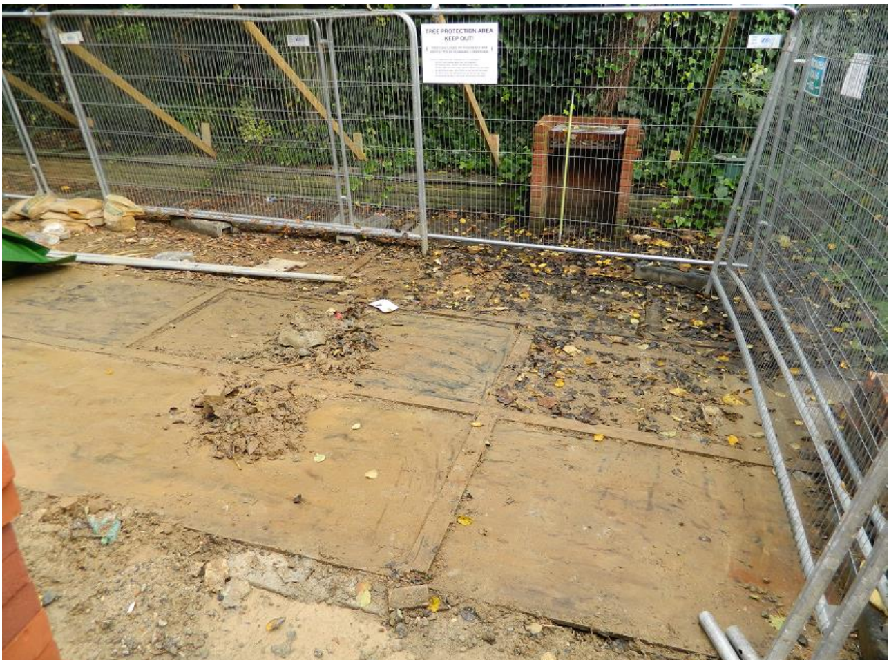
Figure 13. Illustration of ground protection using plywood over existing paving slabs
