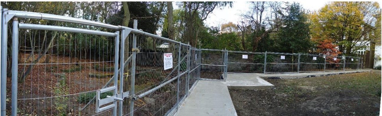
Figure 11. Photograph to illustrate installed protective fencing
