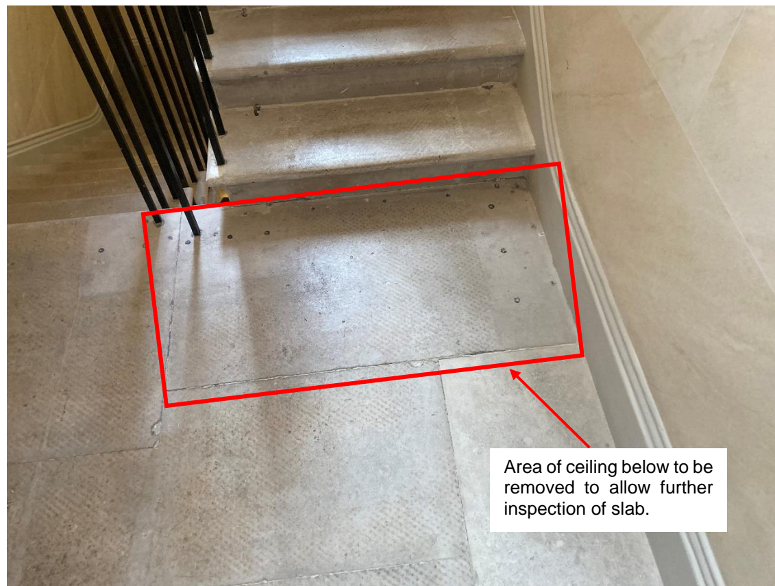
Figure 3: View of first floor landing.
