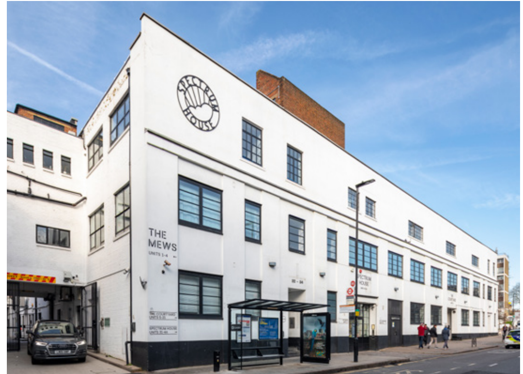
Fig 13: View of the front principal facade of Spectrum House, facing Gordon House Road.
