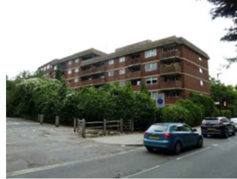
Fig 3: The rear elevation of Salcombe Lodge taken from Gordon House Road.
