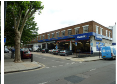
Fig 8: Commercial garage neighbouring Spectrum House to the west.
