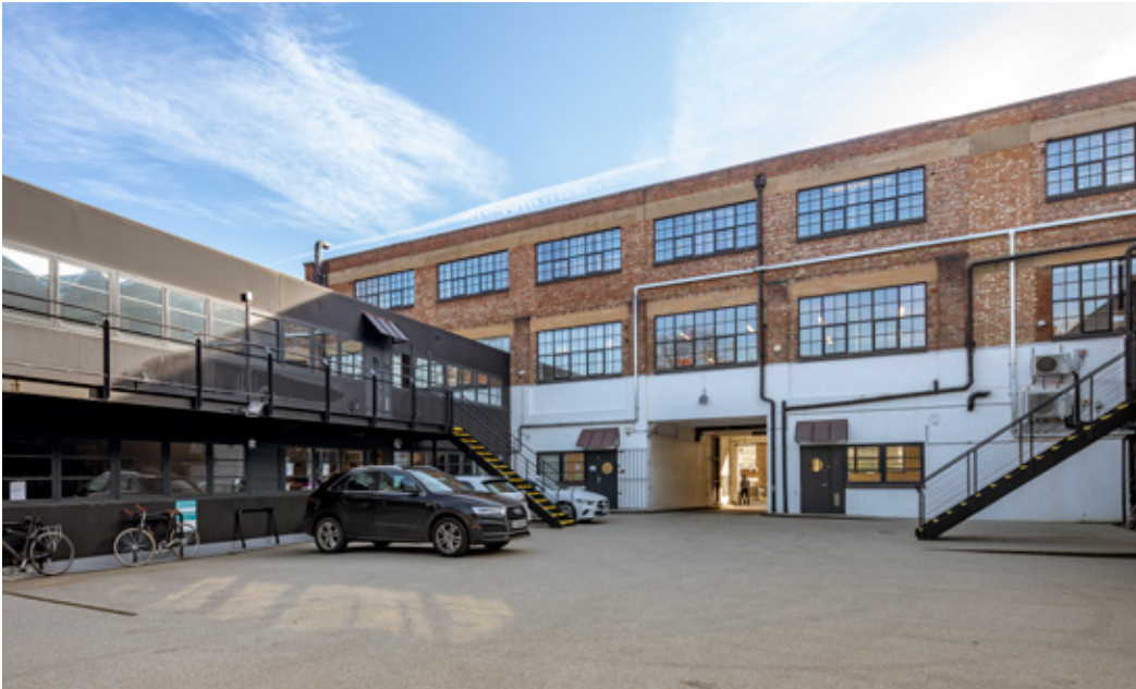
Fig 15: View from the courtyard towards the front three storey elevation.
