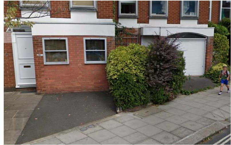
poorly infilled conversion (on the left) and original arched opening to garage to the right
