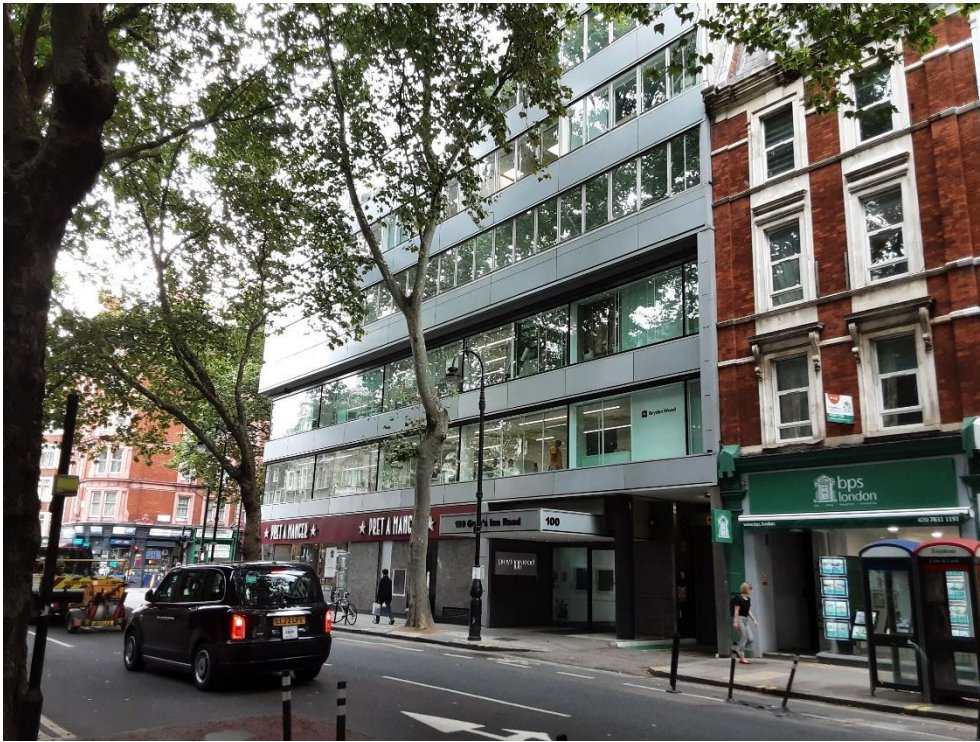
Photograph 1: Building B1 (100 Grays Inn Road)
