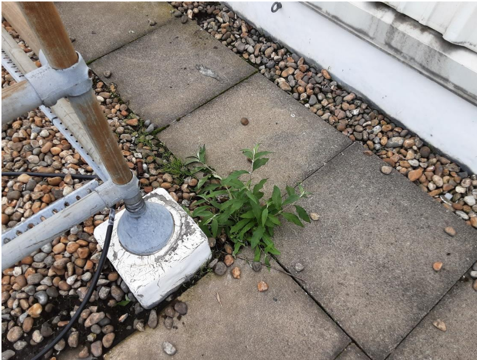
Photograph 3: Butterfly-bush recorded on the roof of building B1 (Target Note 1, Figure 1)
