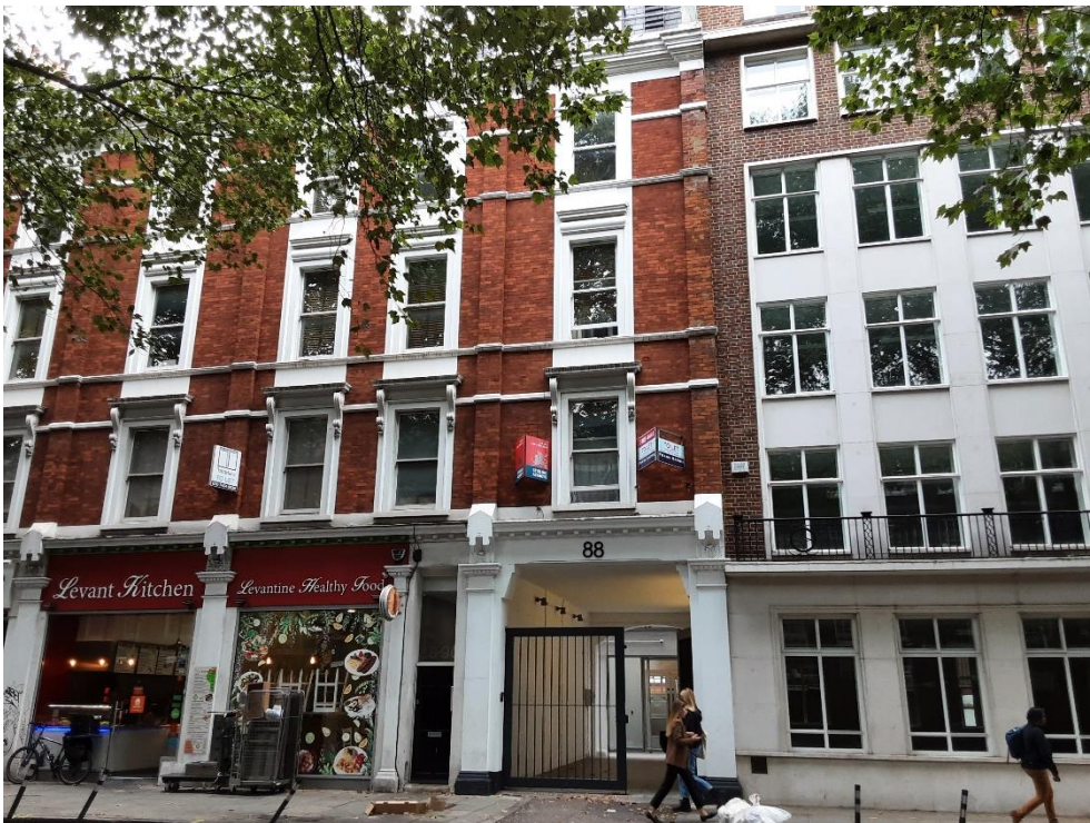
Photograph 2: Building B2 (88 Grays Inn Road)
