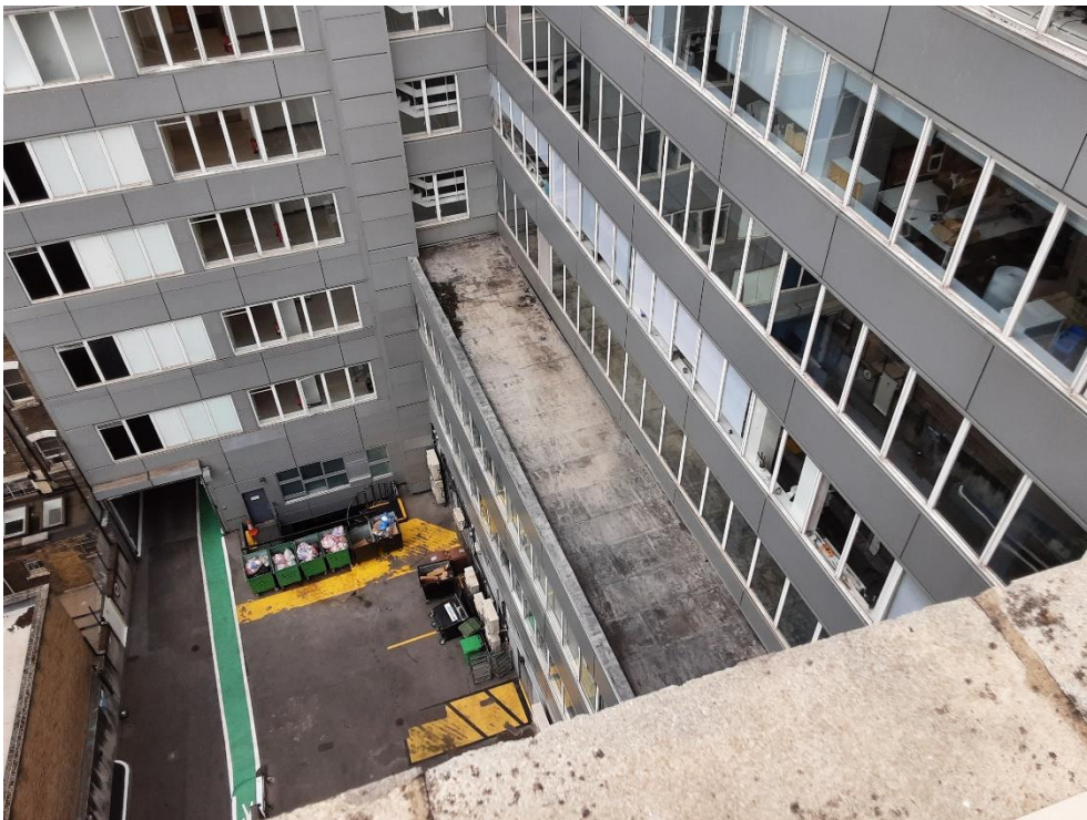
Photograph 4: Area of hardstanding car park and storage
