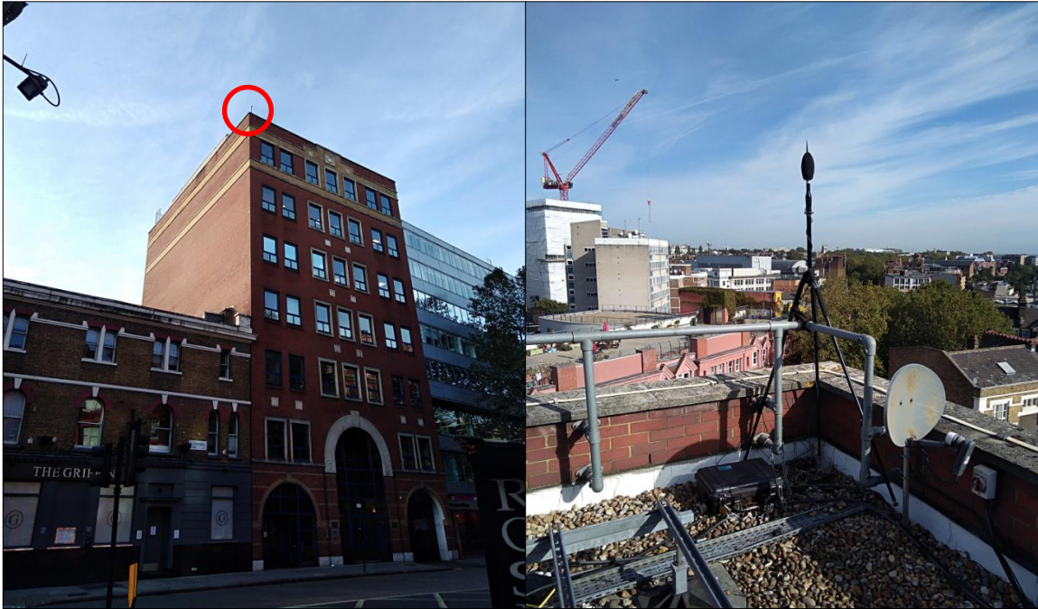
Figure 6 - Photographs showing measurement equipment at location L1 from Clerkenwell Rd and roof perspectives.
