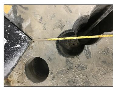
The top of the suspected pile cap was encountered at a depth of 0.46 m, with the base at a depth of 0.7 m.
