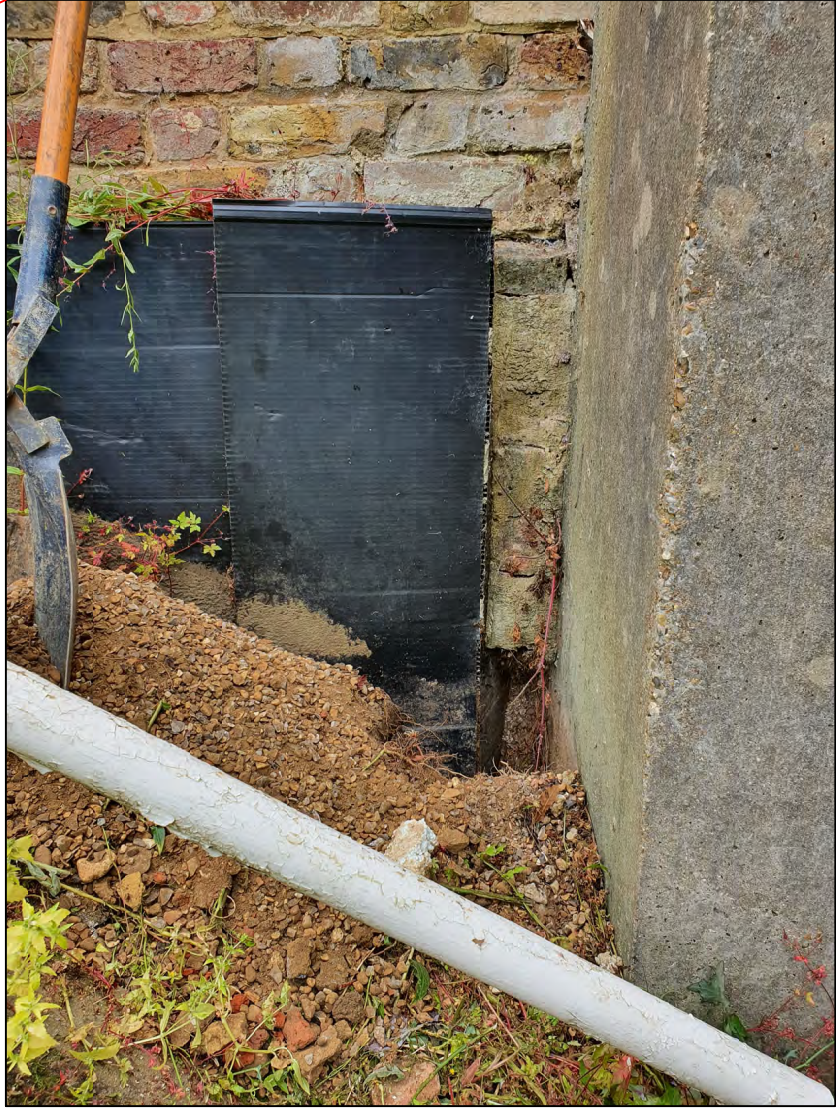
Photo showing intersection of 3 components forming the eastern boundary retaining wall
