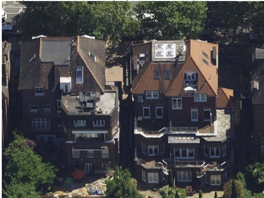
No. 29 Fitzjohn's Avenue (left) and the neighbouring building to the right both have multiple level rear balconies including an inset balcony at roof level
