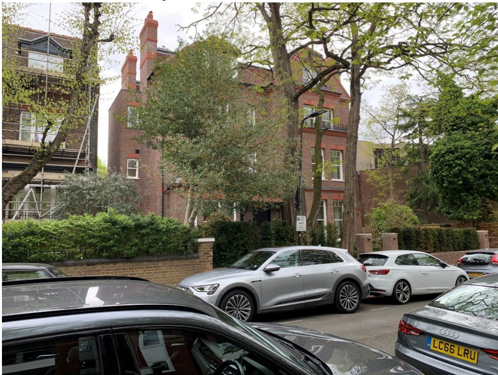
Oblique view towards 2 Maresfield Gardens south-eastward from pavement opposite - terrace / railings not visible due to set back and existing roof form
