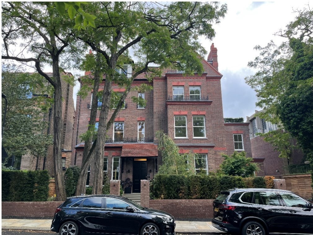
The Site – front / principal elevation to Maresfield Gardens – the proposed roof terrace is not visible due to set-back location behind existing front roof plane – see Proposed Site Section 001_10 for confirmation
