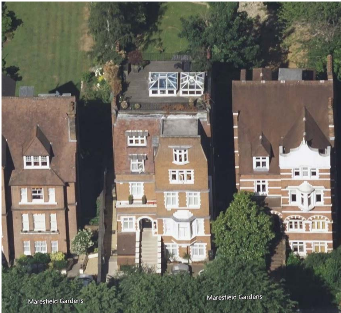
Full width and depth roof terrace located at No.19 Maresfield Gardens with painted black metal balustrade
