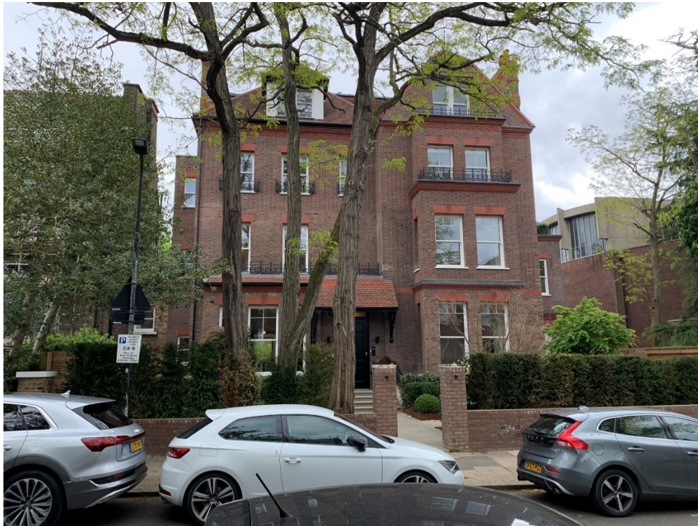
View east towards 2 Maresfield gardens from pavement opposite – terrace / railings not visible due to set back and existing roof form
