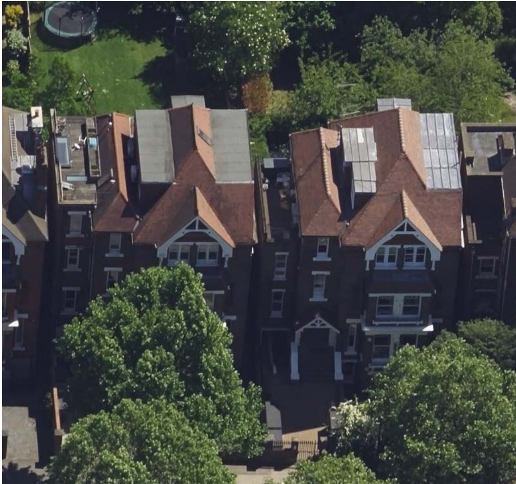
No.10 (left) and 12 (right) Fitzjohn's Avenue – these terraces on the side wings are both visible from street level but positioned so as not to dominate the principal elements of the roofscape.
