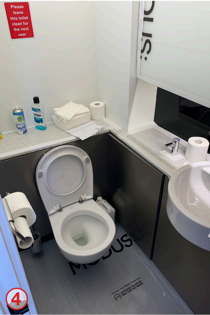
Existing WC facilities.
