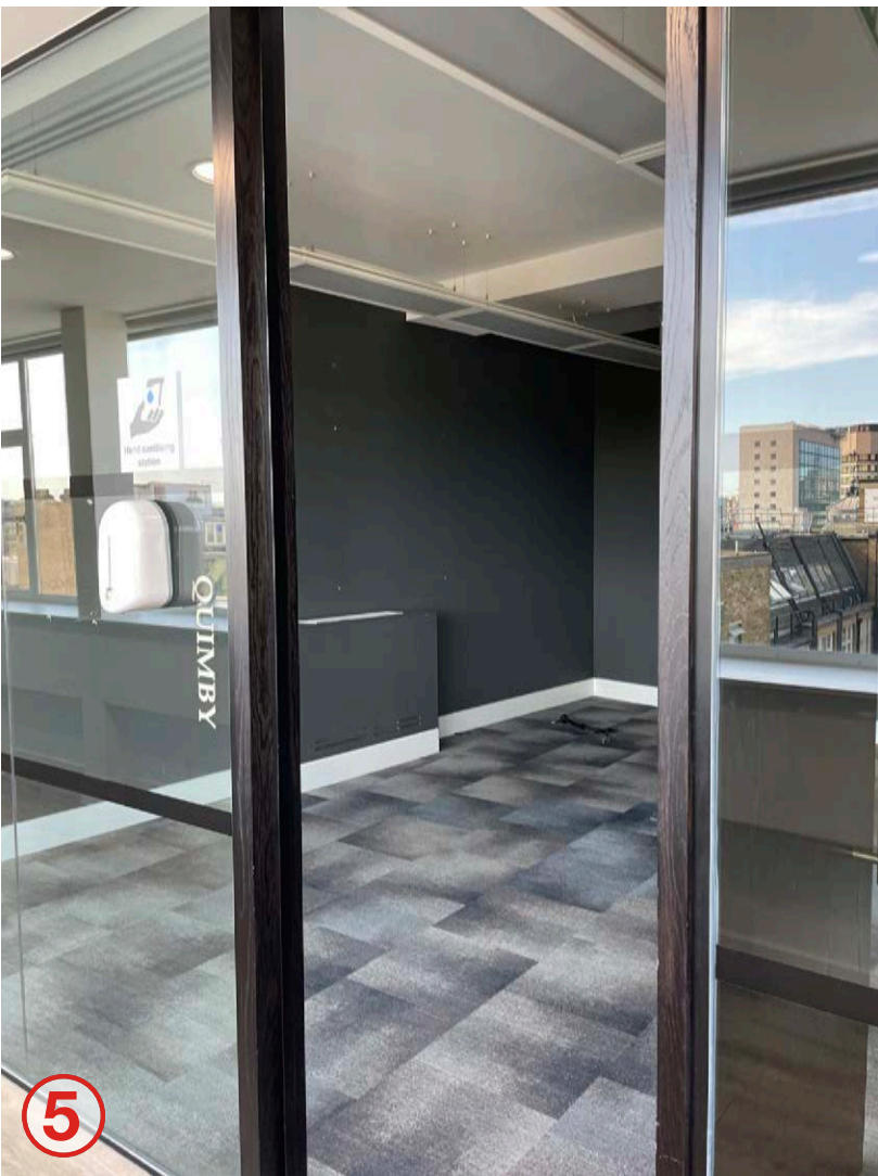
Existing meeting rooms.
