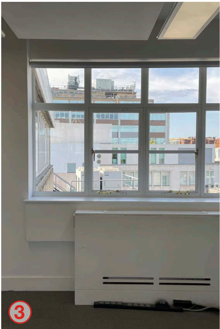
Existing radiator covers.
