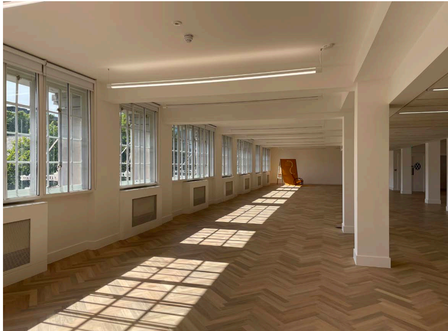
Level 3 office refurbishment in Phase 1.
