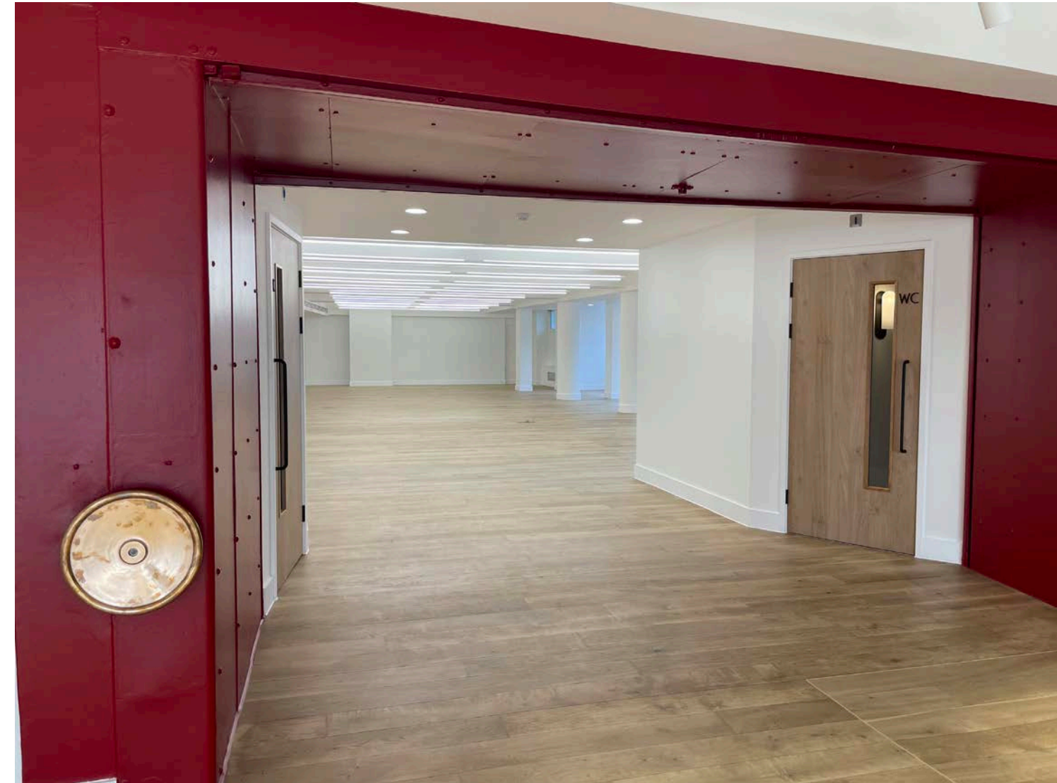
Level 4 office refurbishment in Phase 1.
