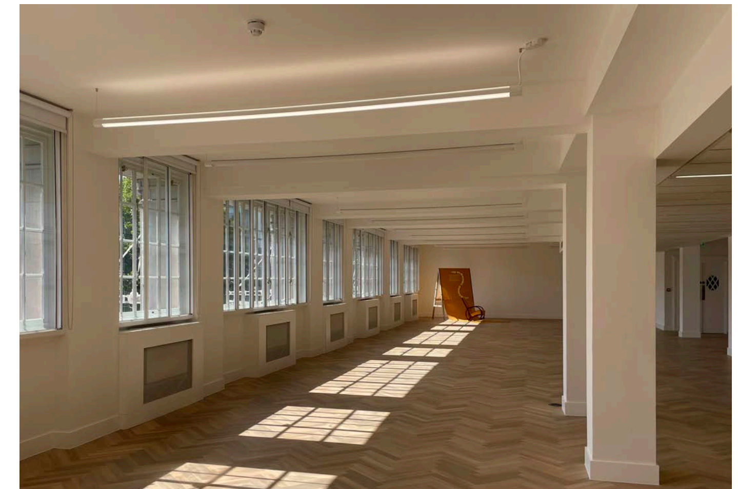
Office ceiling layout at 3rd floor level. Matching suspended LED lighting proposed at 6th floor level.
