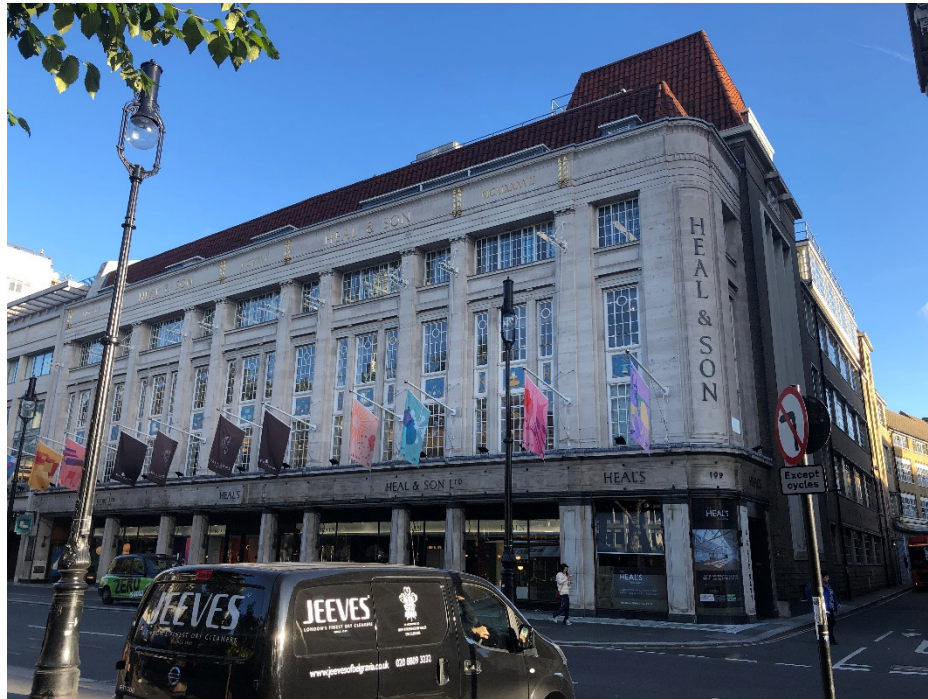
Figure 3.22: The Heals Building Complex looking east at the junction with Alfred Mews
