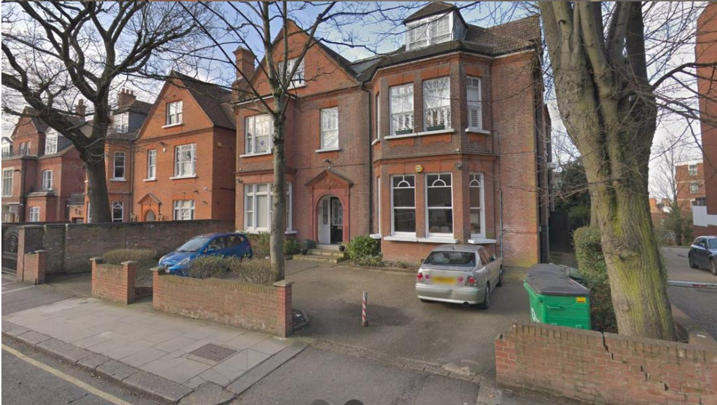
Image 3: Pre-existing front boundary wall
