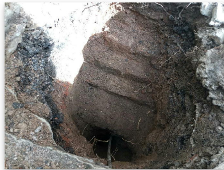
Fig 1.2: Trial Hole 1 Footing
