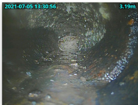
Fig 3.1: Line 4, joint displacement
