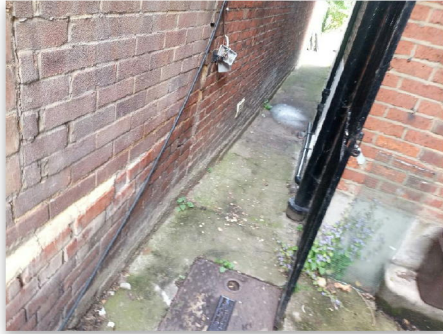
Fig 4.1: Side of property
