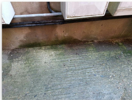
Fig 2.1: Trial Hole 2 Location
