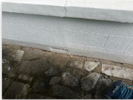
Fig 1.1: Trial Hole 1 Location
