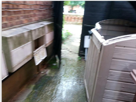
Fig 4.3: Side of property
