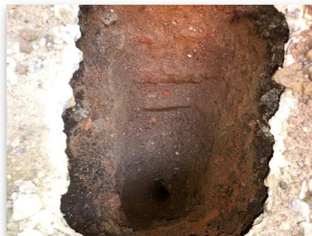
Fig 2.2: Trial Hole 2 Footing
