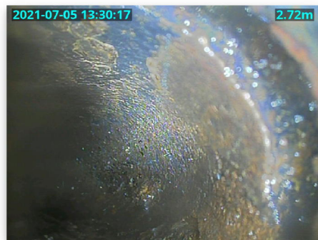
Fig 3.2: Line 4, joint displacement
