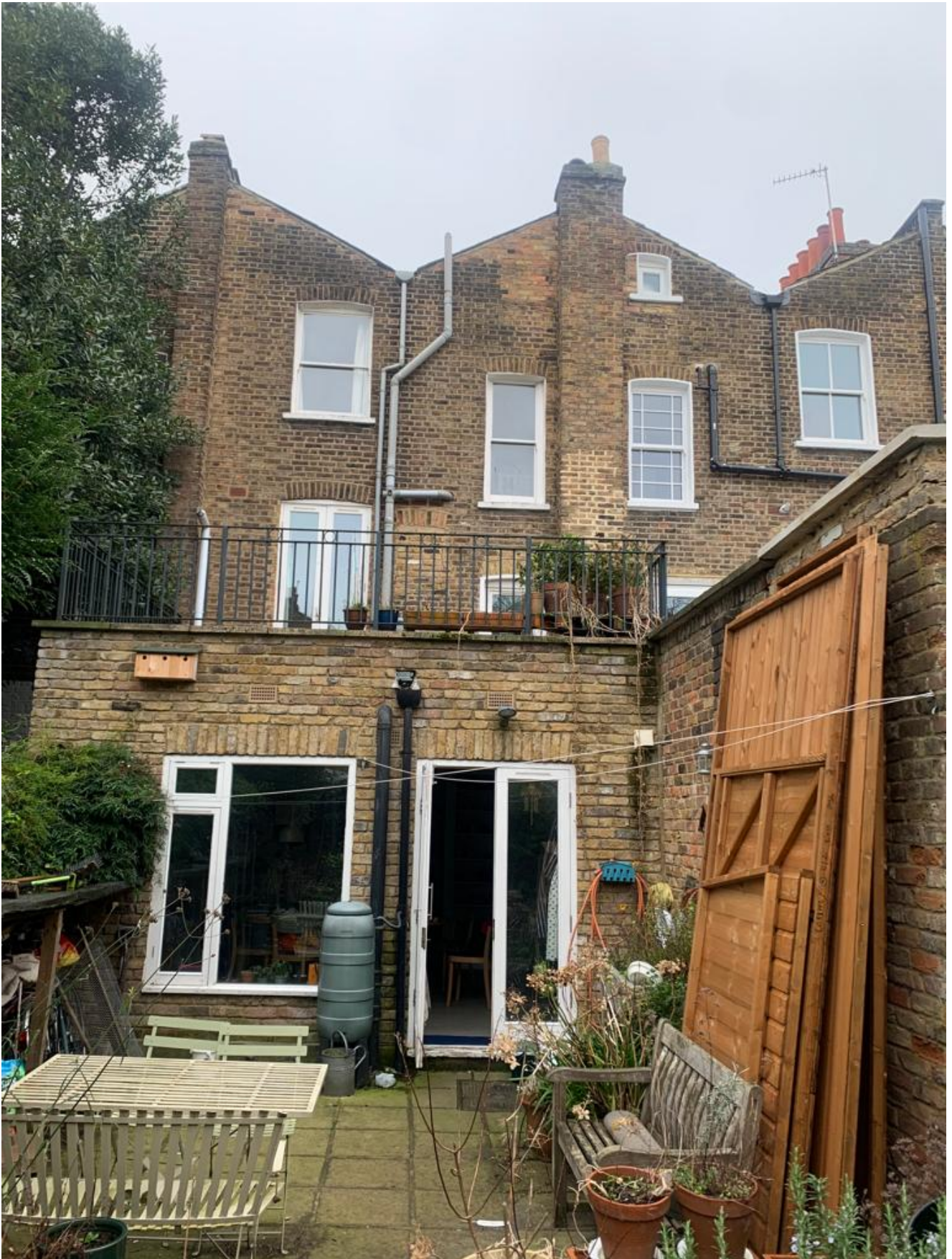
VIEW OF REAR ELEVATION
