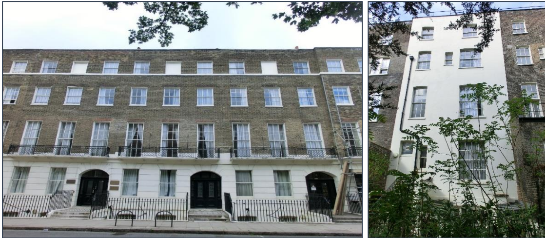
Fig 5 (left). Nos. 4–6 Bedford Place, front elevation. Fig 6 (right) No. 4, rear elevation
