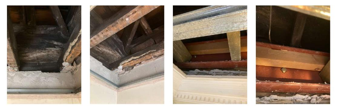
Photos 1-4; No.6 Bedford Place – showing valley-beam and localised valley beam strengthening
