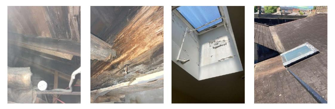
Photos 13; modern (inadequate) sw rafter strengthening and ceiling hanger Photo 14; wet-rot decay of valley beam above number 4 Bedford Place Photo 15 and 16; adjacent roof-light showing source of water ingress
