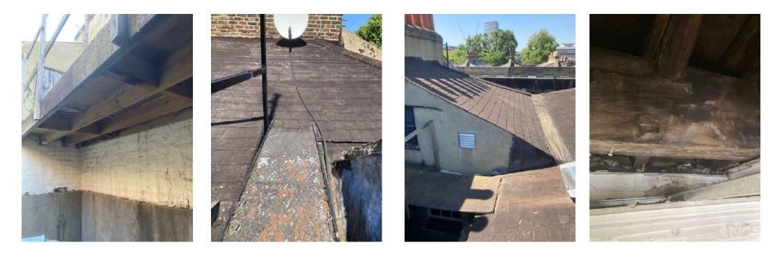
Photos 17-19; various additions typical of all 3 flat-roof areas Photo 20; 4 Bedford Place valley beam showing rafter relationship
