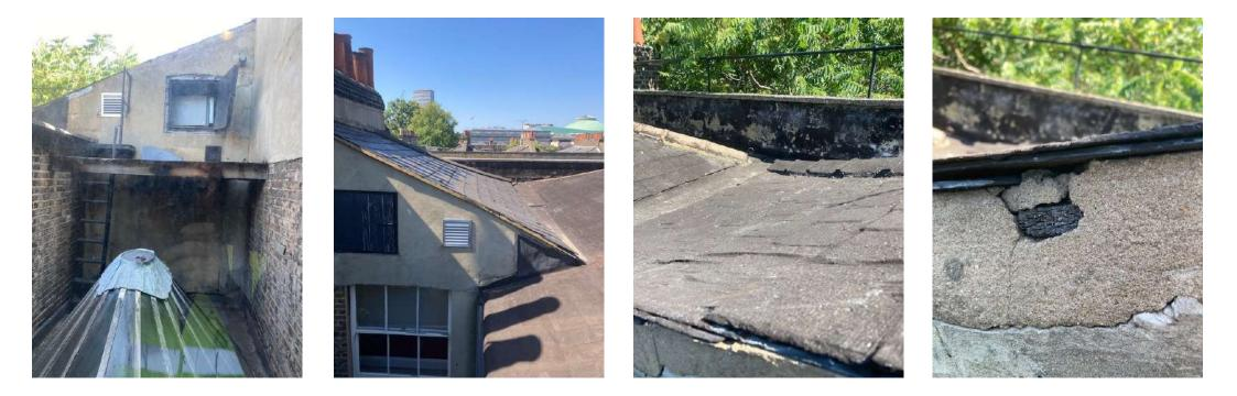
Photos 5; typical flat roof and roof-light feature at 3<sup>rd</sup> floor level Photo 6; typical sagging roof due to overstress of original rafters Photos 7 and 8; asphalt covering across slates
