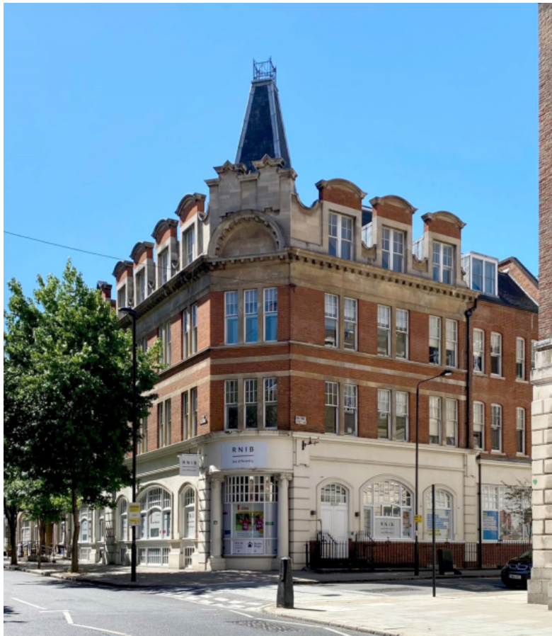
Street view south on Judd Street of existing building
