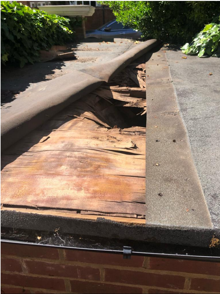
Photo 4 (above): Storm damage to roof of bike shed
