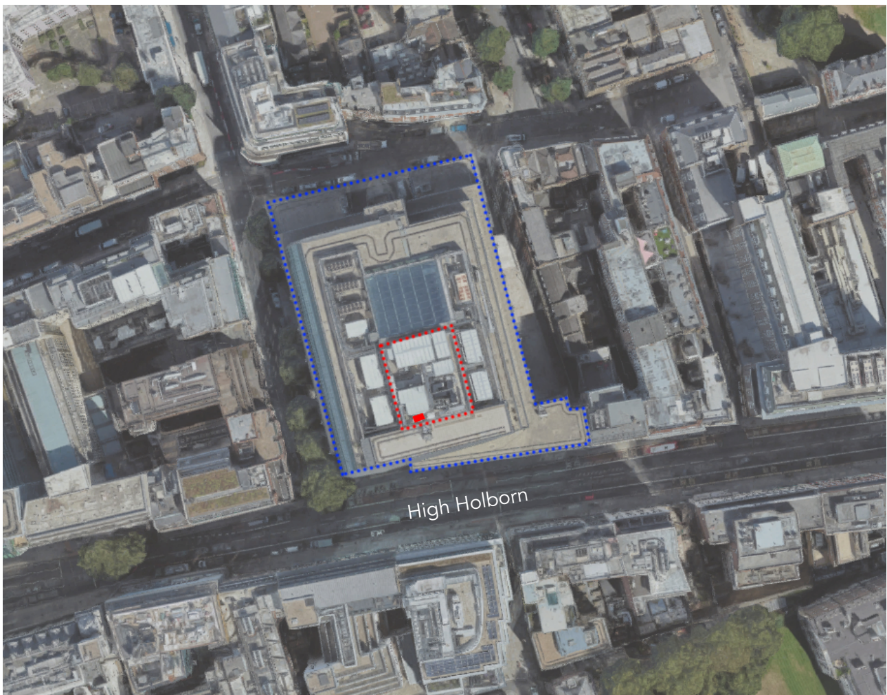
Aerial photo showing hatched in red the proposed location for the new condenser units
