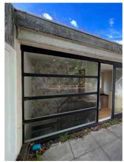
1. exterior fixed terrace window in original finish/colour, unaltered, but in state of disrepair
