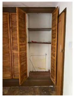
3. original asbestos service void access panel to be replaced with modern equivalent
