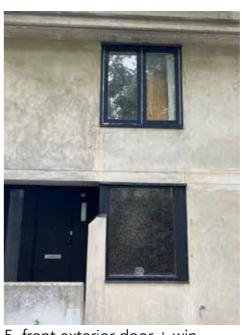
5. front exterior door + windows in original finish/colour, unaltered, but in state of disrepair
