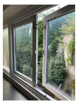
6. original windows painted white internally, and in significant state of disrepair
