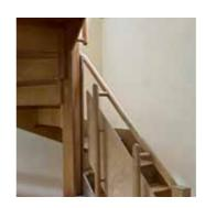
type: original stair material: plywood sanded colour: clear varnish
