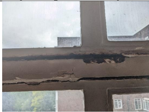
Existing window sill_ weathered and damaged
